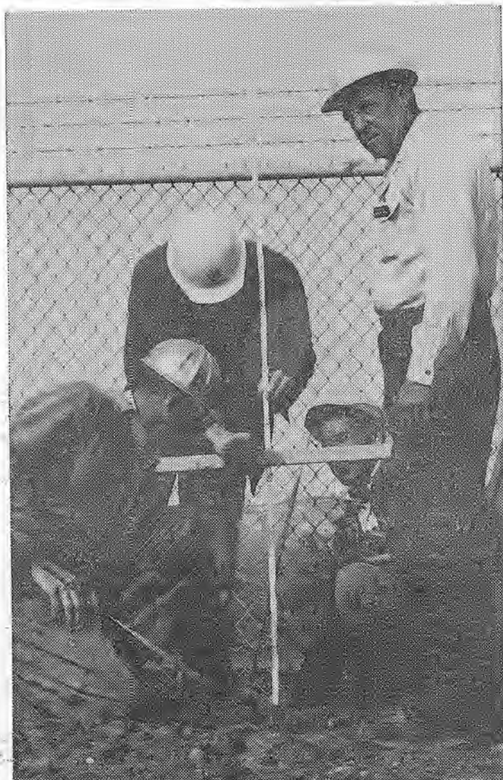
SIGHTING IN . . . Instructor Travis Fodge, right, and grade checkers fix sticks for survey of ammunition dump area.
