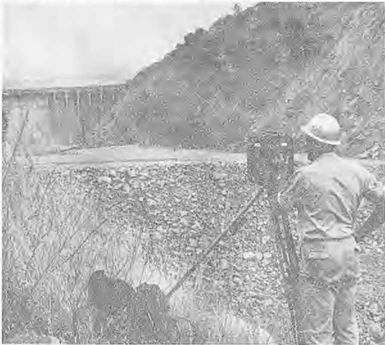
ACCURACY — in Survey work is achieved with this Tellurometer MRA-3 model by the John B. Duff Engineering Survey Co. of San Francisco. Shown here using the electronic instrument on Exchequer Dam east of Merced is Doni Bengston. The MRA-3 has been in use about five years.
