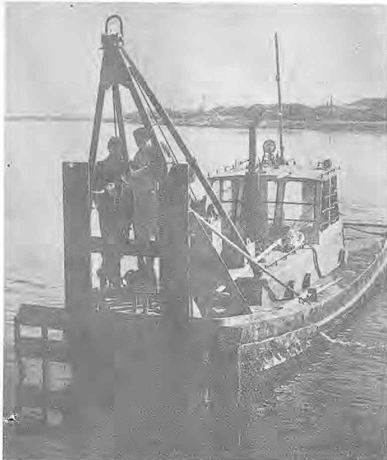
'BOATDOZER' IN ACTION —Here is Brother Terry Murray's "invention" for Hydraulic Dredging Co. Raising and lowering tidal waters determines blade action. (Story below.)
