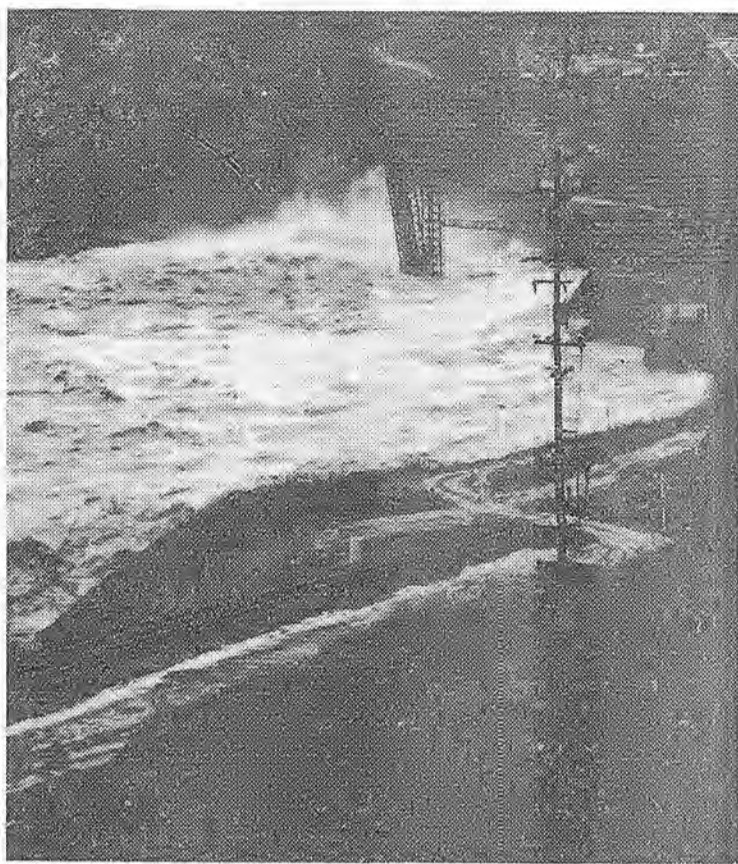
WASHOUT . . . This picture is taken below the Oroville Dam and shows the Frazier-Davis Construction Company's Bailey Bridge just before the water coming from the two diversion tunnels washed it out.
