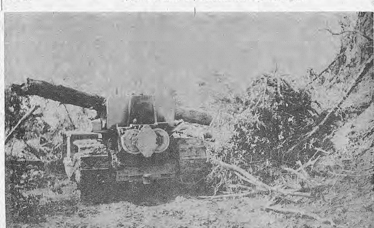
**THIS WAS** a fatal accident in the Sacramento area. The operator of the cat was killed by a falling tree—because the cat did not have a strong cab over his head. Any work in clearing should be done with equipment that will protect operators from this danger.
