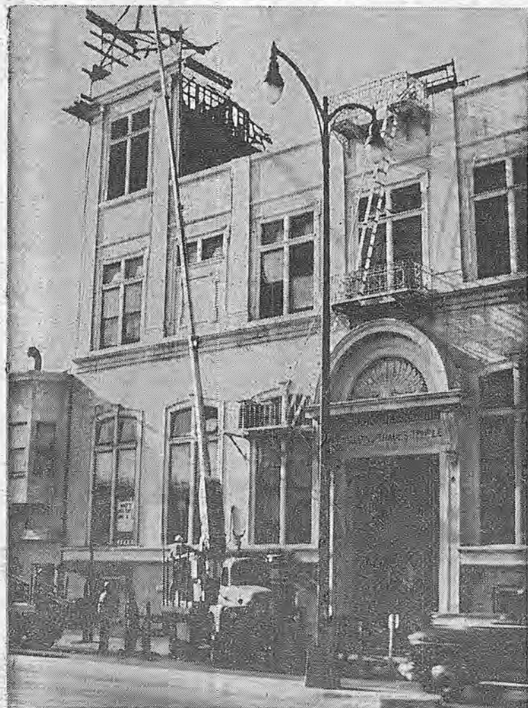
TOP COMING OFF —Aftermath of the San Francisco Building Trades Temple fire left surprisingly little damage visible outside the lower stories. In this photo a crane is shown removing the last of the debris of the burned-out third floor. With a temporary roof, the Temple is now a two-story structure.
