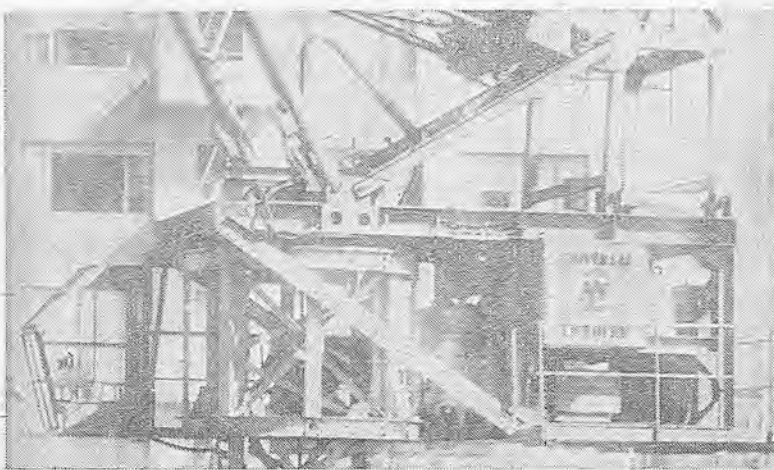
Close-up of cab section on giant crane erecting new apartments on SF's Nob Hill. Note glass cab out front with control levers. Operator really has a front seat.
