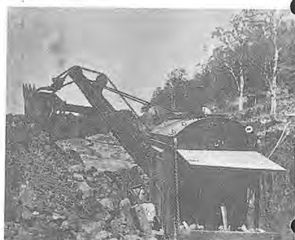
EARLY SHOVELS —Back in 1911, this was the type shovels used on various California dirt jobs. The buckets look like two-yards, and notice chain over shivs. Jobs were at Battle Creek and St. Helena.
