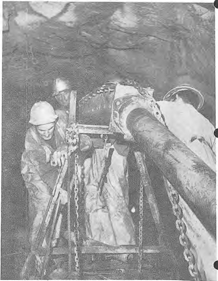
STRAINING —teamwork, headed by Brother Bob Kaine, left, steward on Emil Anderson Auburn Tunnel, helps dismantle this slick line. Auburn tunnel is part of 24 miles of tunnels in a system to carry American River water to arid sections of Placer County.
