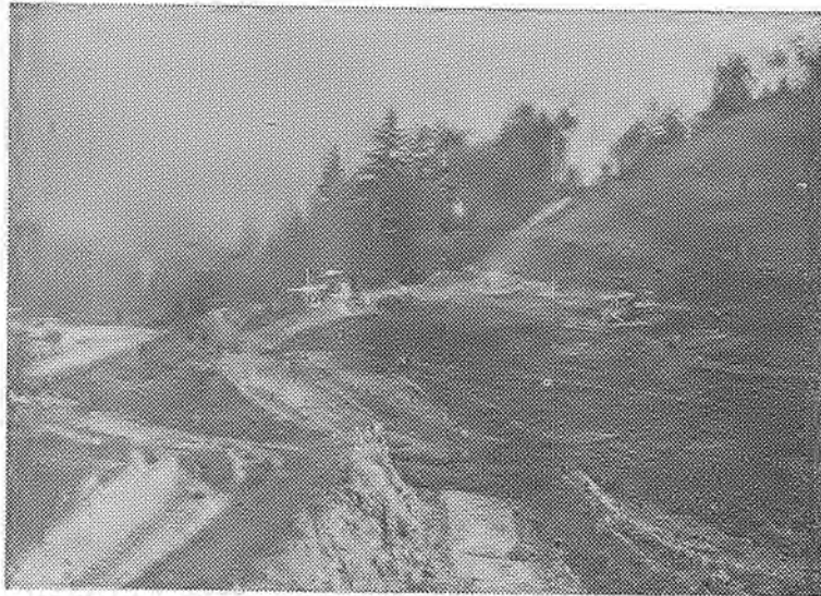
SLIDE REMOVAL —it happens every year in Eureka. They are the first to be flooded and first to have trouble with slides. Here equipment works to cleanup a 160,000 cubic yard slide at Willow Creek last year. Crews have a 310-foot cut on three benches and moving 500 yards hourly.
