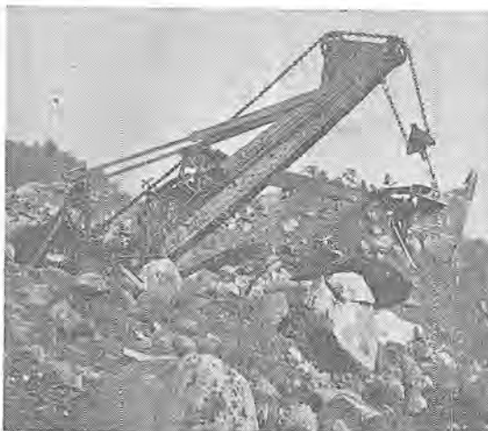
EARLY SHOVELS —Back in 1911, this was the type shovels used on various California dirt jobs. The buckets look like two-yards, and notice chain over shivs. Jobs were at Battle Creek and St. Helena.
