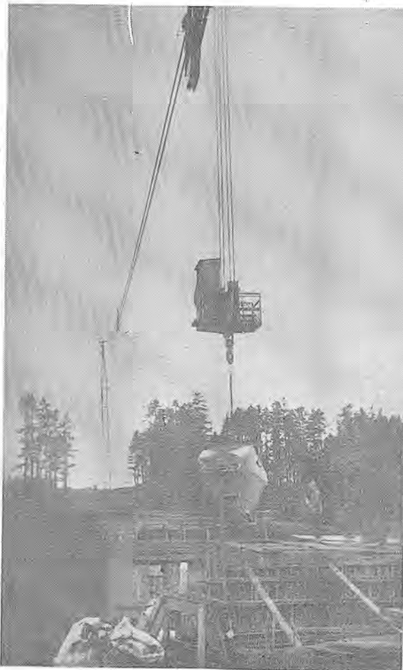
HIGHLINE — Operating Engineers erected this highline to erect a bridge near Casper, Calif. in the Redwood Empire. The booms are 180 feet high
