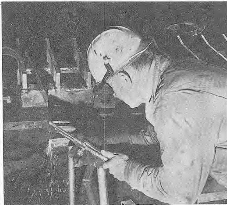
CUTTING, FITTING —Carl Earl is shown here in Industrial Service shops cutting angle iron for small brush rake in back-ground. The company is one of few making brush and rock rakes.
