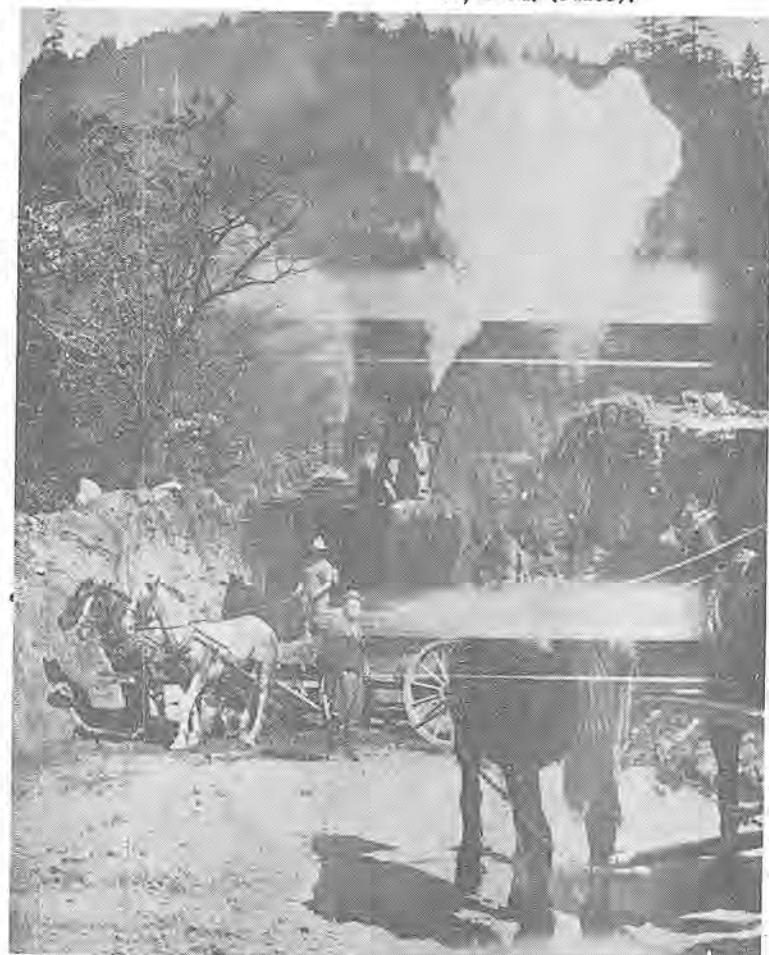
OLD PUFFER —this old steam shovel, operated by Ed Arhardt in foreground, loaded "Western Dump" wagons on St. Helena Rd. above Calistoga.
