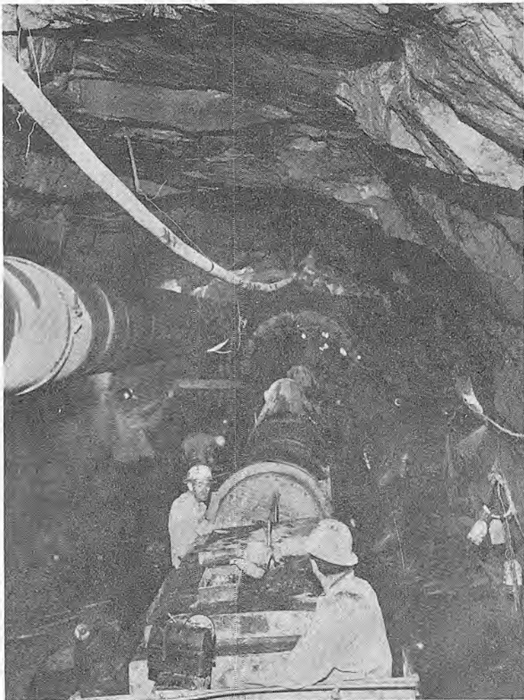
INSIDE —Auburn Tunnel workmen do final cleanup before end of shift. Here is dinky train hauling concrete for lining tunnel on Emil Anderson Co. job. Project was finished 18 months ahead of schedule, a record for overall Middle Fork projects.
