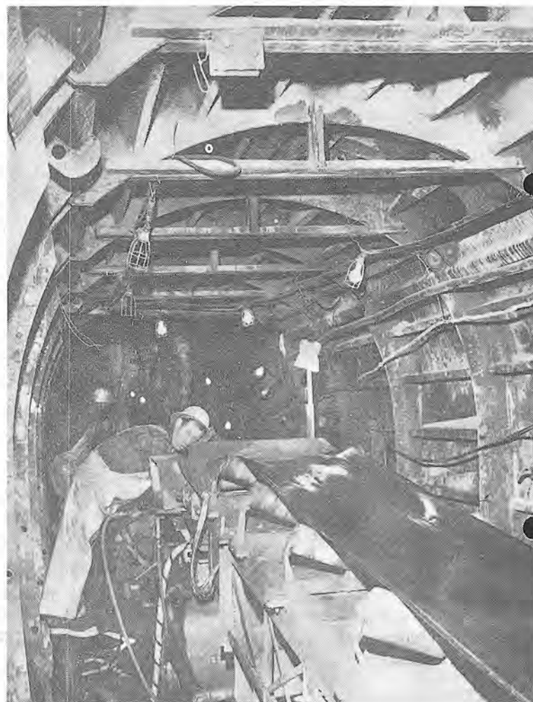
CLEANUP —Brother Bill (Squeaky) Ash cleans press-well in Auburn Tunnel which connects American River and Auburn Ravine in Cphir, a distance of 17,758 feet under the city of Auburn. This was last tunnel in county's Middle Fork American River project.
