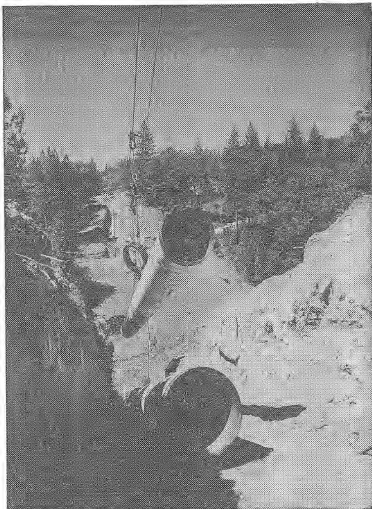
HIGH WIRE ACT . . . this 40-foot section of pipe, weighing 3000 pounds, sails through the air from Indiana Creeks to canyon rim during construction of Dobbins-Oregon House Canal. Pipe rides aboard carriage on highline system, a wire rope attached to one side of canyon and a winch on the other side.
