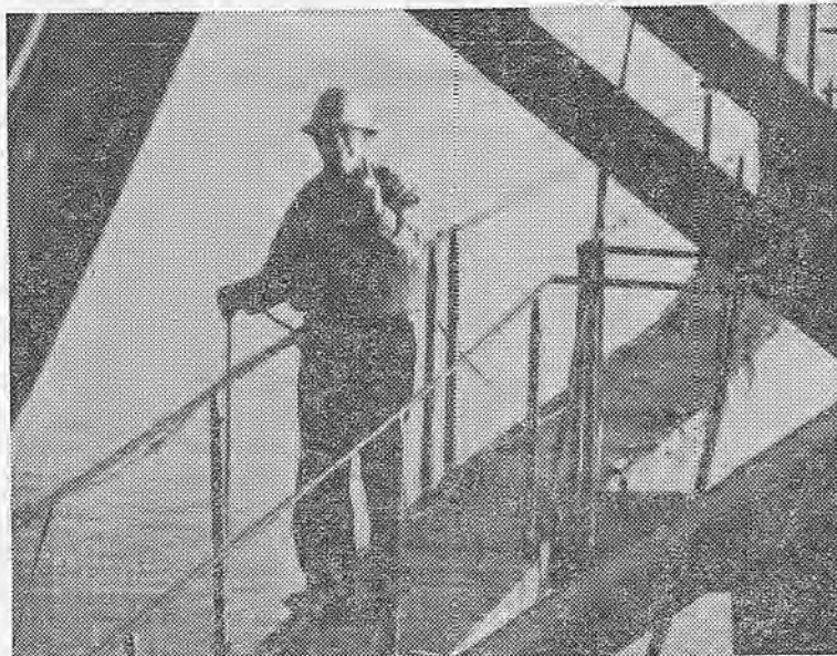
ONE FINGER UP is the hand signal for 31 feet, as Gene Sullivan, deckhand on the Papoose, takes sounding out on the catwalk over the area where the dredge's hydraulic intake head is churning up the bottom of the deepwater channel and pumping away the muck. Gene is also a 25-year member of the union.
