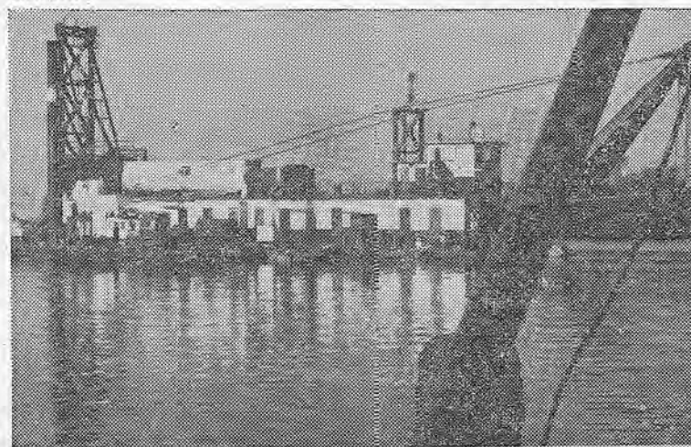
IT GOES IN HERE: The hydraulic dredge Papoose is shown here at work in a stretch of the deepwater ship channel where a plug has just been cut through, in the Cache Slough area. The A-frame boom controlling the suction intake is at the front (right). Several hundred feet of flexible-jointed pipe on pontoons carries the muck away at the rear (left). Three shifts man the dredge on a 24-hour basis.
