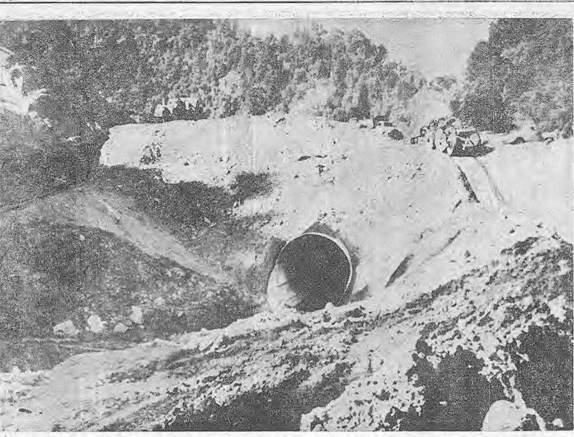
**NO MORE FLOODS** at Longvale. Arthur B. Siri and Carey Brothers have finished placing a 9-foot pipe in the trouble area. They first removed a slide and afterward rebuilt the hill.
