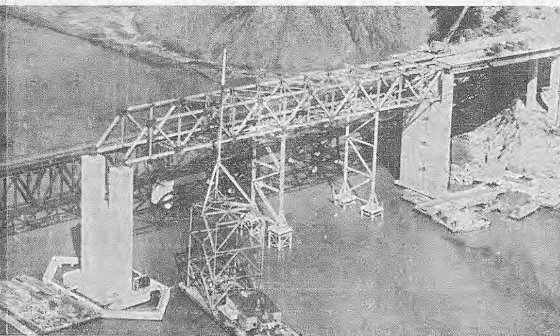
**JUDY ANN and DANIEL C.** are at work on the Benicia-Martinez Bridge. Judy Ann (right) sets steel on the 429-foot first span. The rig can lift 100 tons, but the biggest lift on this span was 63 tons. The tower is 78 feet with a 30-foot mast, a 100-foot main boom plus 20-foot jib and a
