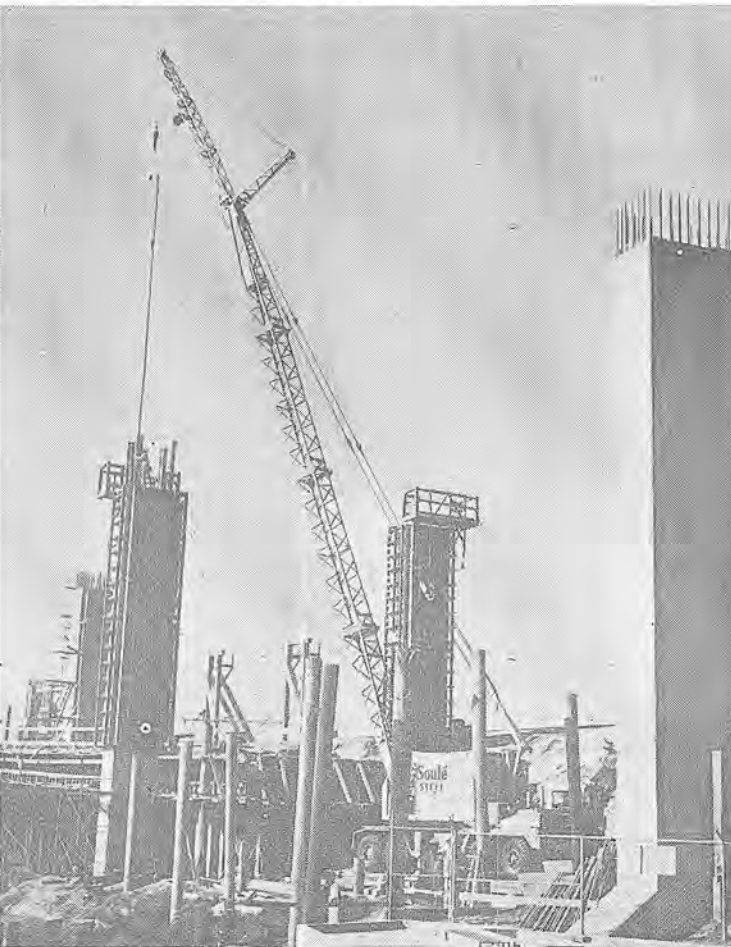
NEW FREEWAY —Guy F. Atkinson Co. has started the south San Francisco freeway, and shown here is Soule Steel's truck crane placing reinforcing steel in pillar. Note workman at top of pillar.
