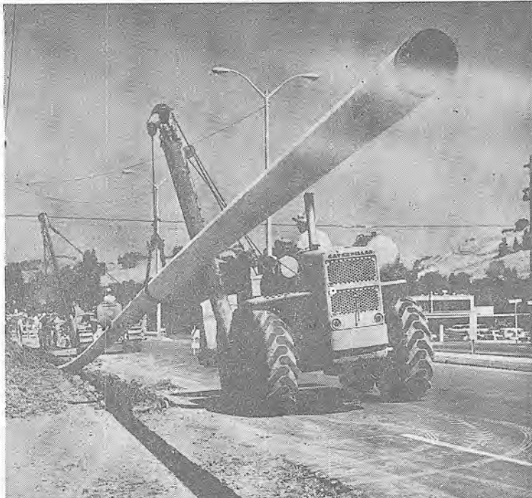
PIPELINE —job for Shell Refinery for its new Contra Costa addition is providing work for Laco 3 men. Shown here is a 130-foot section being placed in trench along street near Lafayette. Pipeline will end at Oakland Municipal Airport.
