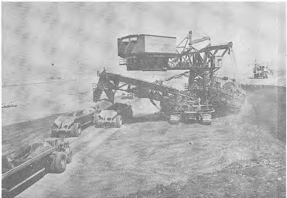
DIGGER —the San Luis Dam "wheel" is still churning away after nearly two years of continuous operation. Here it is shown biting into bank at one end while loading trucks at the other.
