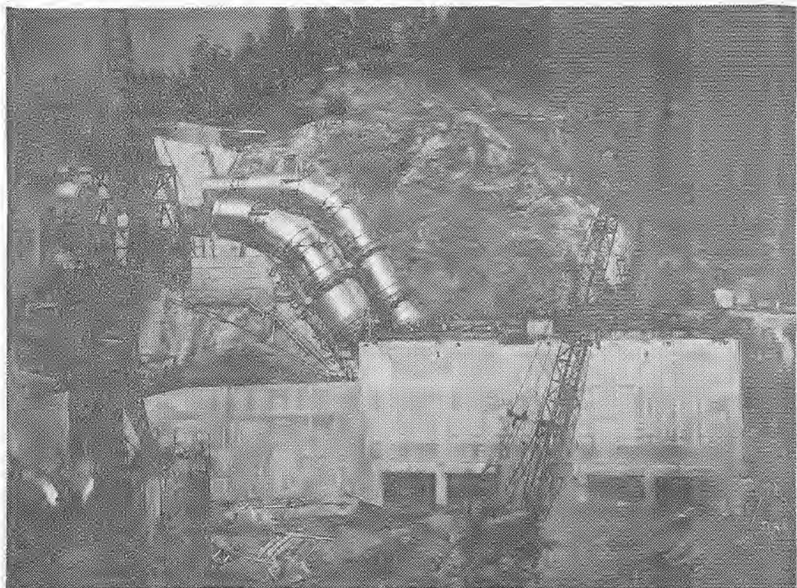
McCLOUD POWERHOUSE —on the Pit River, about half a mile upstream from Pit 5 Powerhouse, will have a capacity of 155,000 kilowatts installed in two six-jet vertical shaft impulse water generating units supplied with water from Iron Canyon Reservoir. The excavation for the penstock is in the background.
