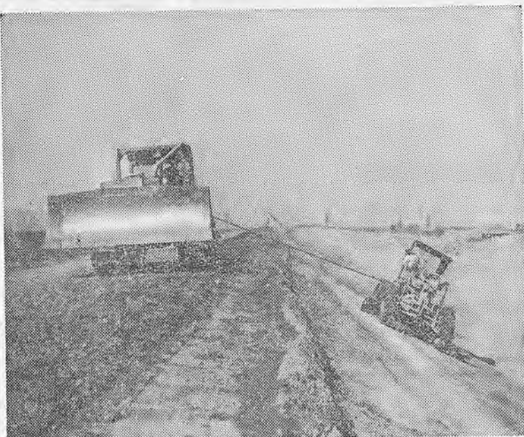
ON THE SLANT: Secured by a cable to the rig on the bank, Brother Wynn Wood is cutting back slopes with his blade on Gibbons & Reed's Weber Canal job.
