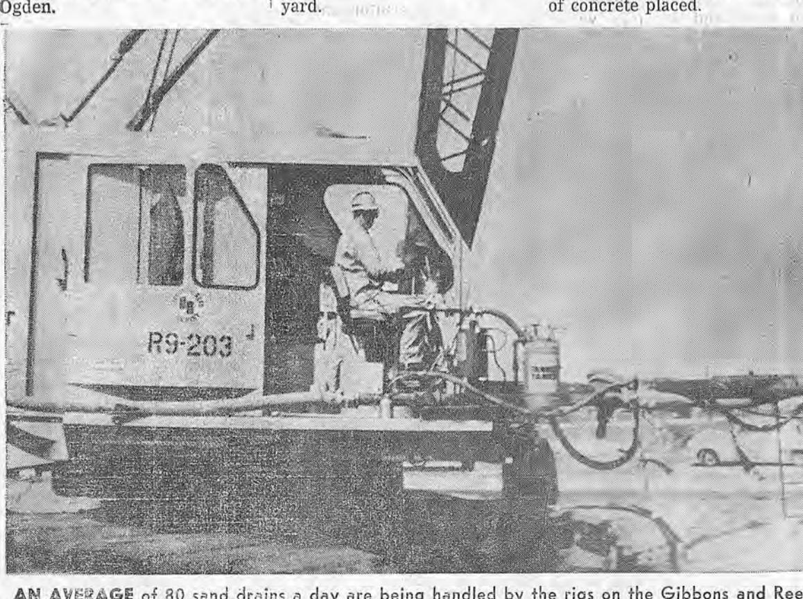
**AN AVERAGE** of 80 sand drains a day are being handled by the rigs on the Gibbons and Reed freeway job at Salt Lake. Parrel Didrickson is at the controls on the day shift and Red Fenner is the operator on the second shift.
