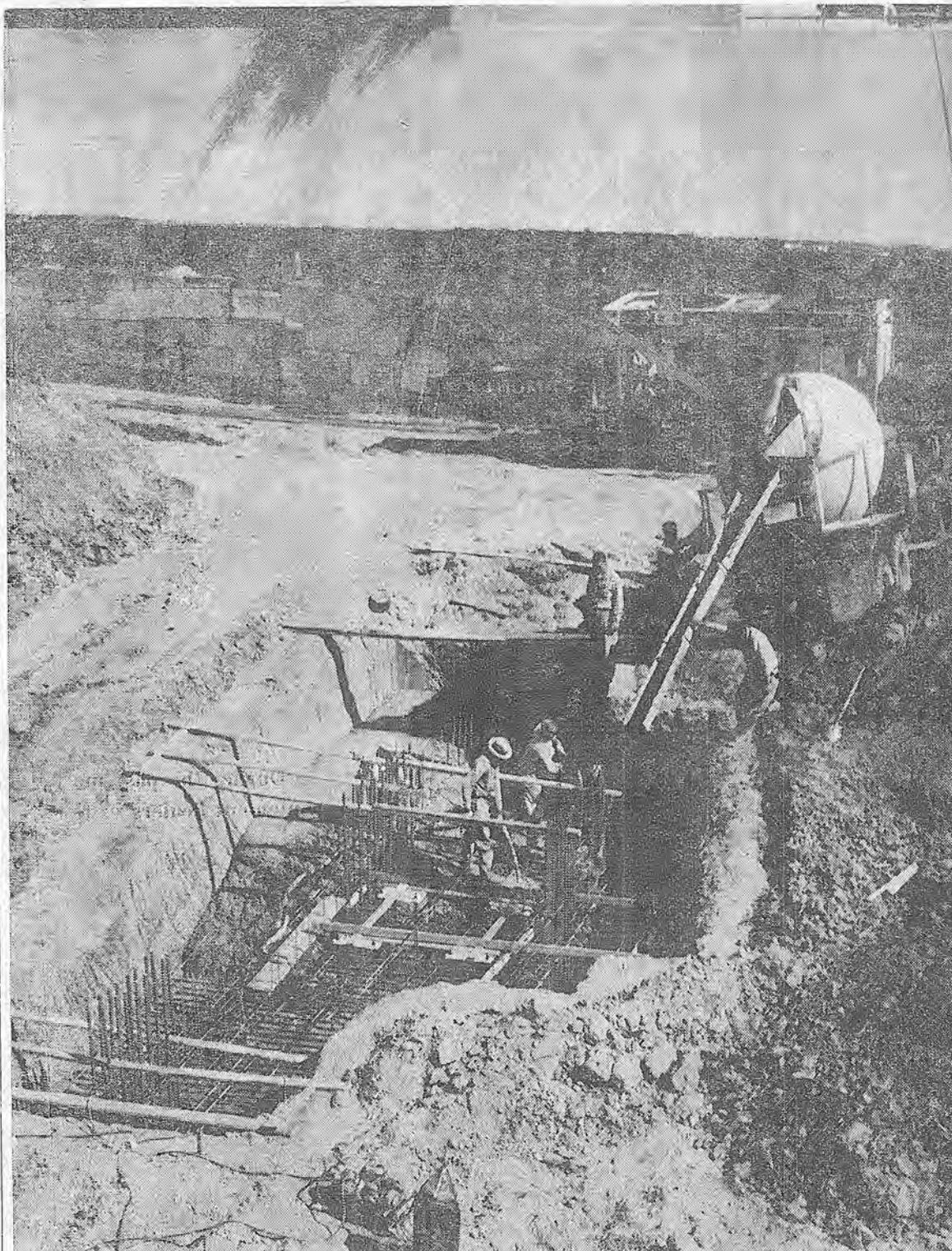
**FIRST STEP** in construction of the Fontana apartments in San Francisco was installation of the "walking" cranes. Foundation is shown being poured for one of the two cranes that were familiar sight on the San Francisco skyline during construction of the Comstock on Nob Hill. Erection of the Fontana itself will follow the crane installation. As one floor is finished the cranes are raised for the next floor.
