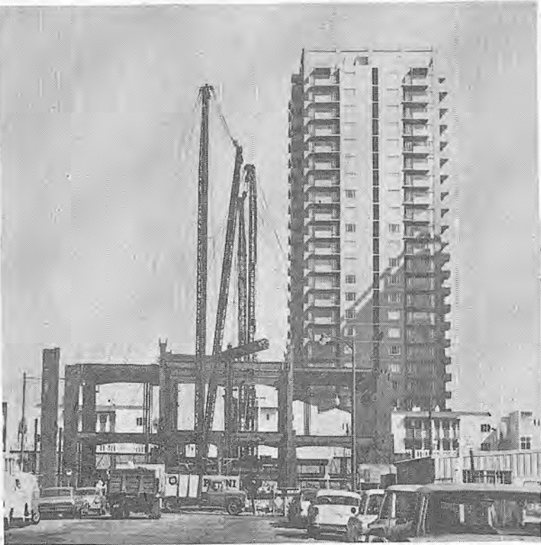
GOING UP —San Francisco is building toward the sky, and shown in above pictures is evidence. At top Operator Ken White is setting forms in place on south freeway. Below, two guyed derricks, 40 and 70 tons each, are placing red iron on phase 2 of Golden Gateway project.
