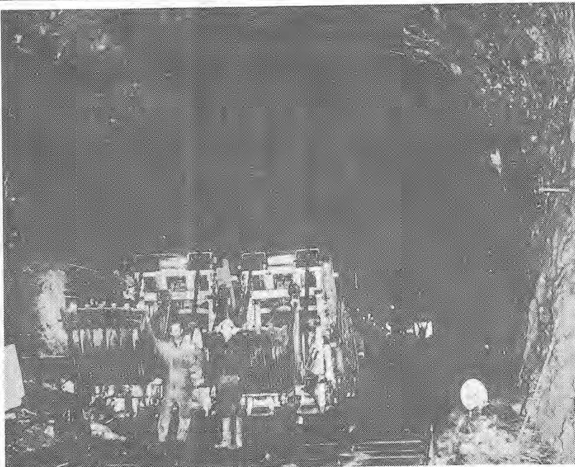
NEW ZEALAND . . . the tail race tunnel on South Island here is rushing along with this 100-2 Conway mucker on the Manipouri Power project, according to Brother Jim Powell, now a service representative for Goodman Manufacturing of Chicago, Ill., owners of all patents on this machine.
