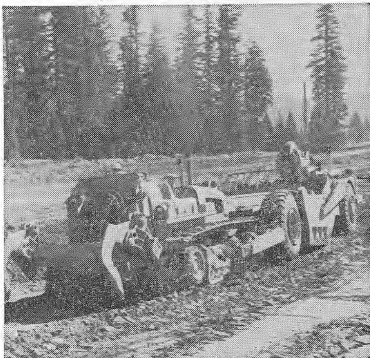
AT LAKE ALMANOR: Photo shows a T.C. 12 Euclid dozer and 631-B Cat scraper working on the Morrison-Knudsen job at Lake Almanor Dam, which is now just about wound up.
