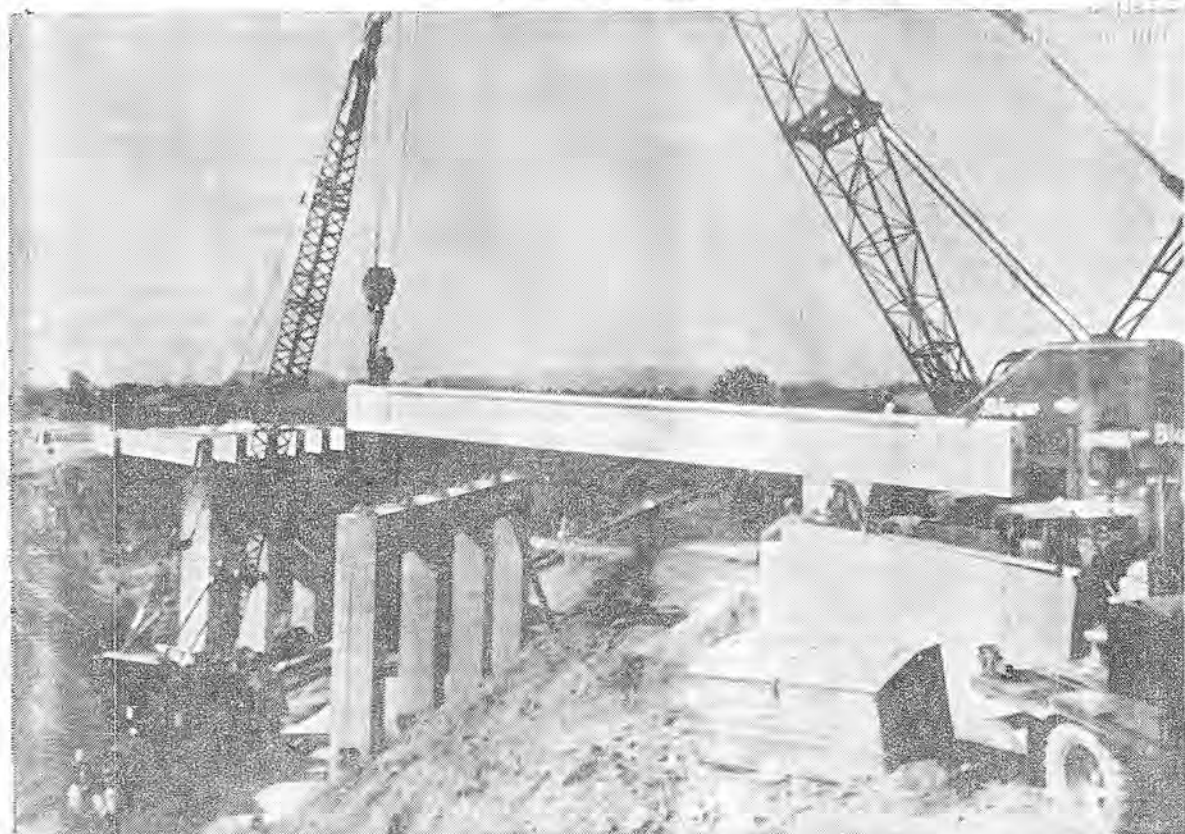
WORK PROGRESSES on the railroad overpass of the freeway north of Santa Rosa. Bigge Construction is working the beams. Guy F. Atkinson has his men on single shifts on this job and on the freeway job at Ukiah.
