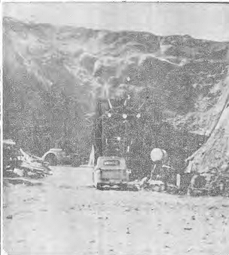
CONCRETE will be poured soon on Case-Hood and Foster's diversion tunnel at the Black Butte Dam job.
