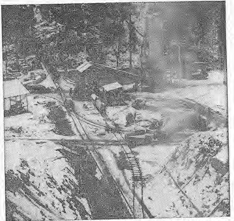
WINTRY SCENE . . . at the P. G. & E. McCloud-Pit project near Redding. Dry mix batch plant is set up outside Portal 6. Motors travel between Portals 6 and 7 at bottom of picture.
