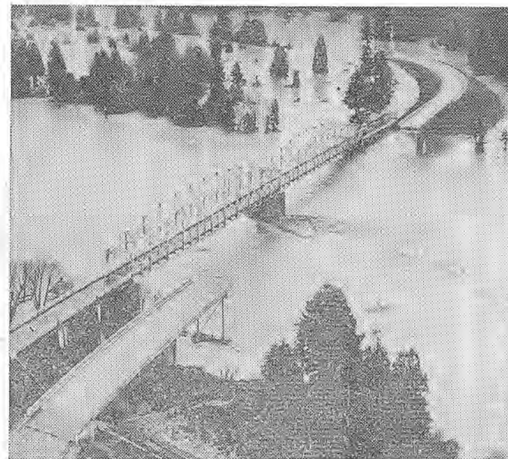
ONE DOWN . . . the recently completed southbound Scotia bridge on Hy. 101 was washed away by high water, which at its peak covered both bridges. The old bridge at left is standing.
