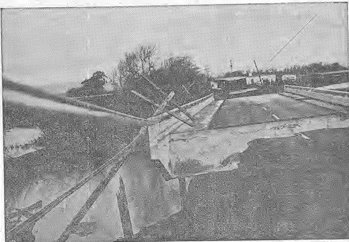
DISLOCATED . . . this bridge at Arlynda Corners, near Ferndale, was jarred loose from its mooring as raging river washed footings away. Note electric pole leaning to left.
