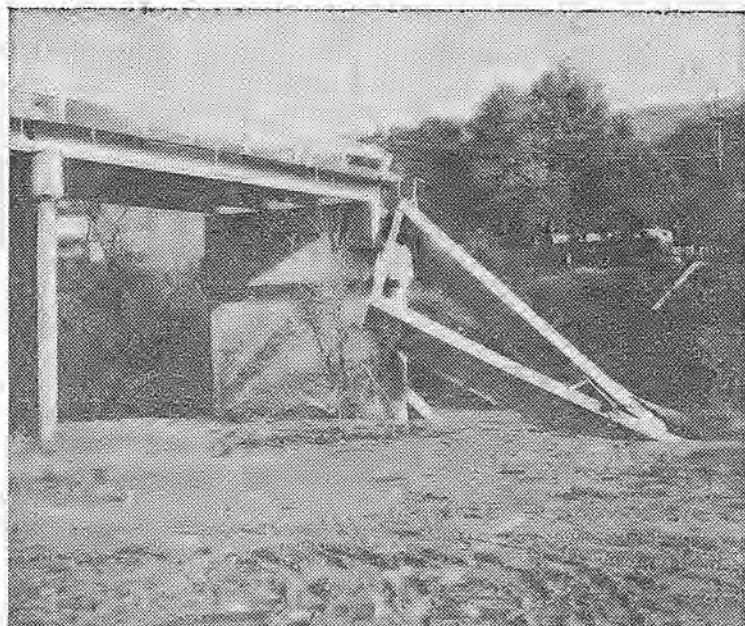
TWISTED BRIDGE . . . torrential waters washed away and undermined this vehicle bridge near Calpella in Mendocino County, isolating and stranding hundreds of persons and interrupting highway traffic in the vicinity.
