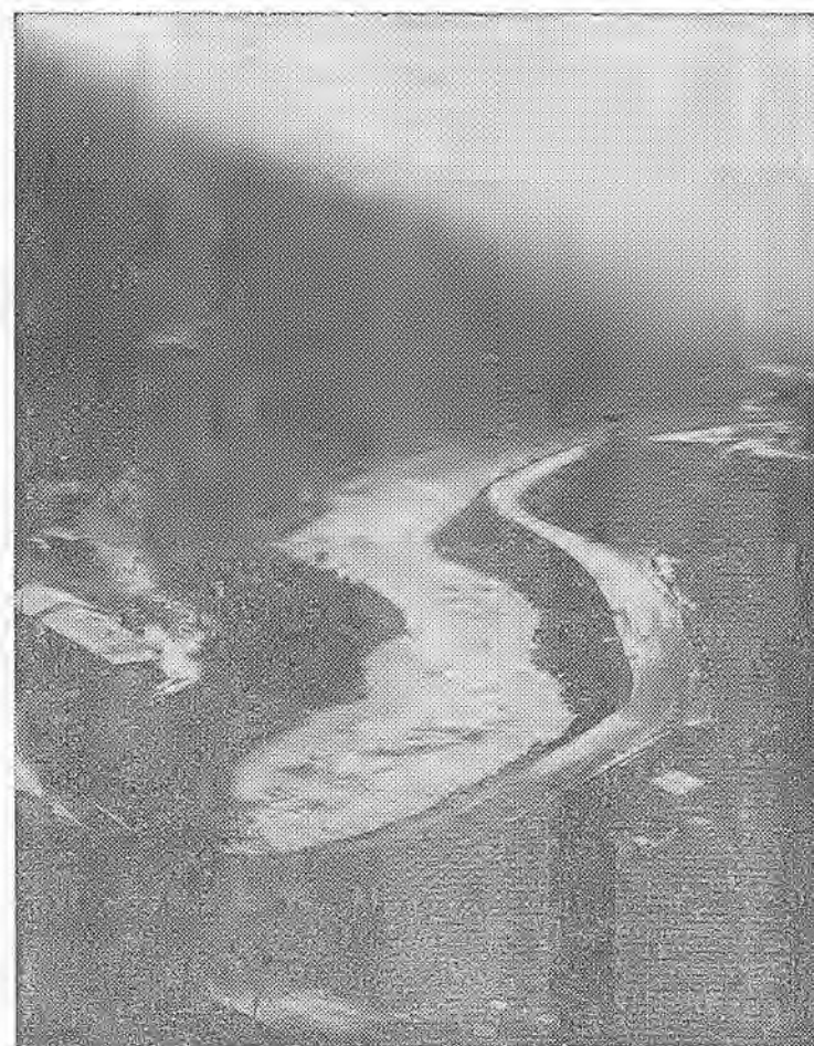
STORM . . . heavy rains washed away coffer dam below Pit 7 on McCloud-Pit project, inundating powerhouse, batch plant and stockpile, and construction sheds to left.
