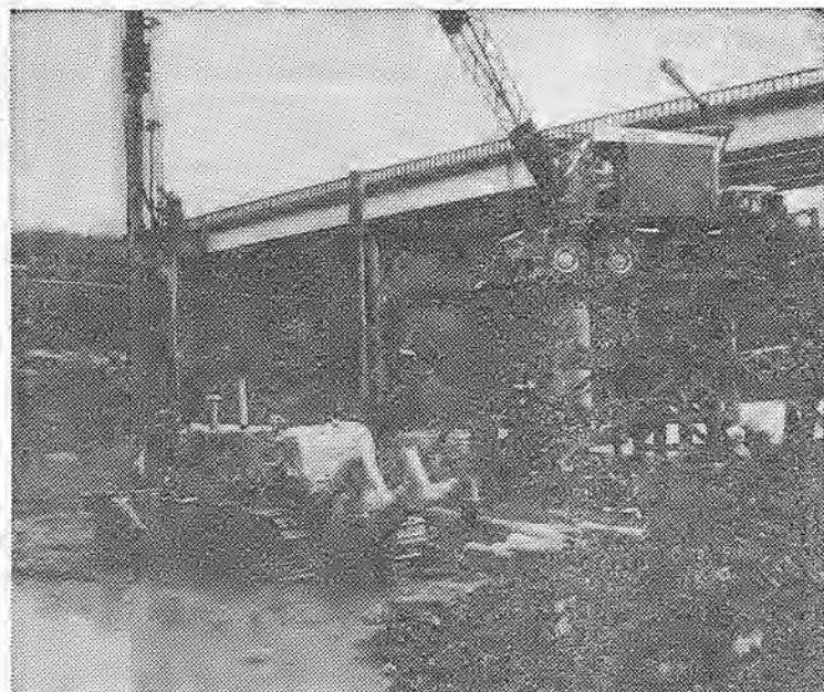
EMERGENCY WORK . . . railroad bridge near Calpella, Mendocino county, was washed out. George Carr Co. is repairing it with Brothers Everett Sasser, Charles LaDelle and Earl Wallace on the equipment.
