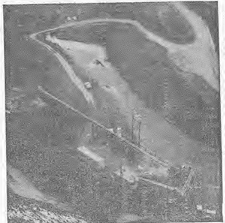
STOCKPILE . . . this portable crusher and conveyor is placing impervious material for Kiewit & Sons at McCloud Damsite. Bridge is left center was washed out 9 days later by floods.
