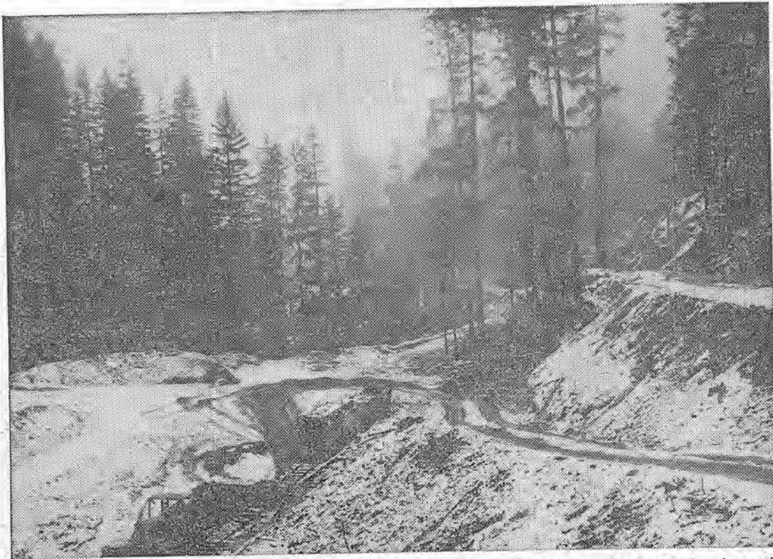
SNOWBOUND . . . construction roads to Hawkins Creek were dotted with heavy haul trucks and stalled vehicles. Fog shrouds most of area shown here, while a scraper churns away leveling muck hauled out of Portals 6 and 7 at McCloud-Pit Project.
