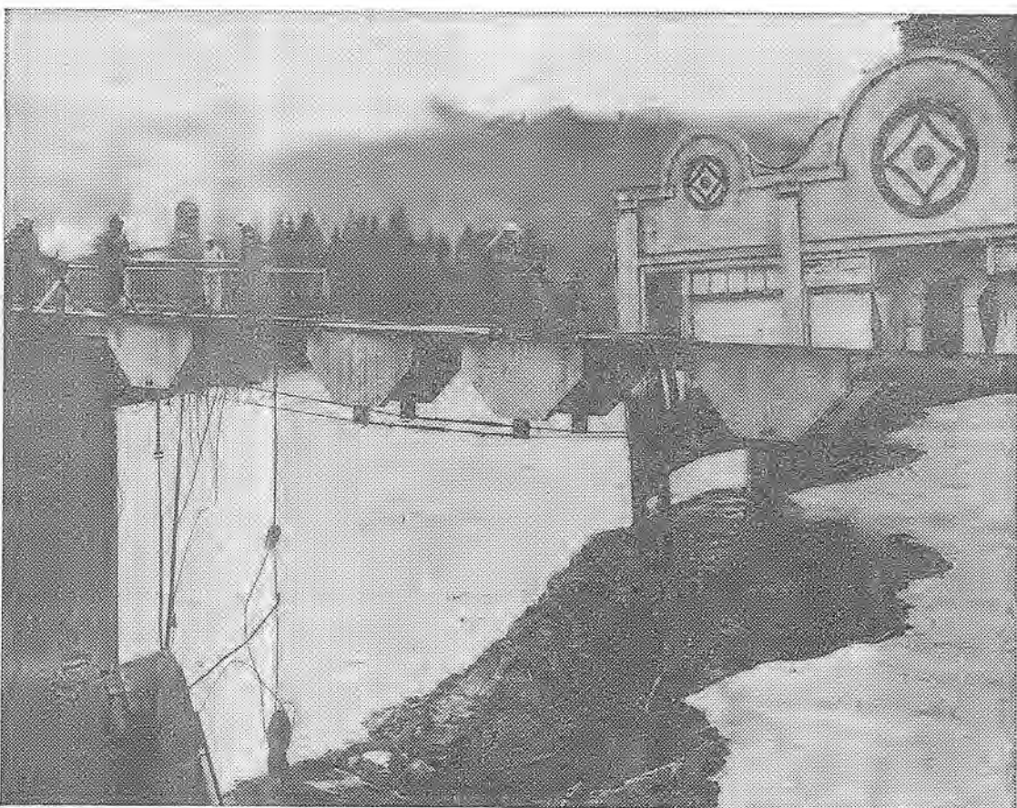
TIGHT ROPE . . . engineers place catwalk foot bridge at Rio Dell as Eel River undercut bank washed out Scotia bridge. In background is a bakery building teetering over river.
