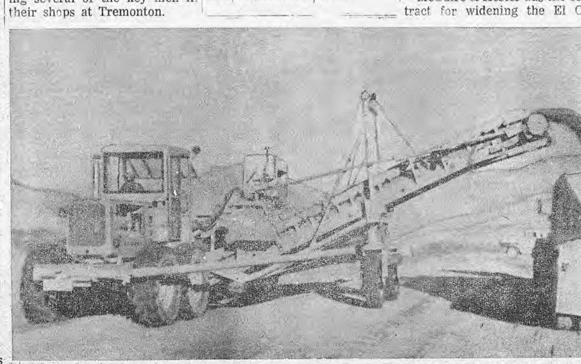
THIS "JEBCO" LOADER, owned by Gibbons and Reed Company and with Joel Williams operating it, is mounted on a "cat 14" blade with a loading capacity of 500 yards per hour. The "loader" is a conveyor belt that can be dropped from blade in one hour. The loading speed is about four miles per hour. The conveyor has its own engine for power.
