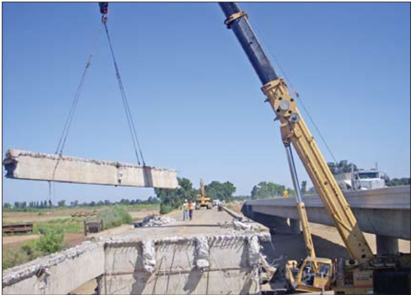
Crane Operator Chris Honomichl with General Crane lifts 30-ton concrete girders from the old bridge spanning the Merced River near Snelling.
