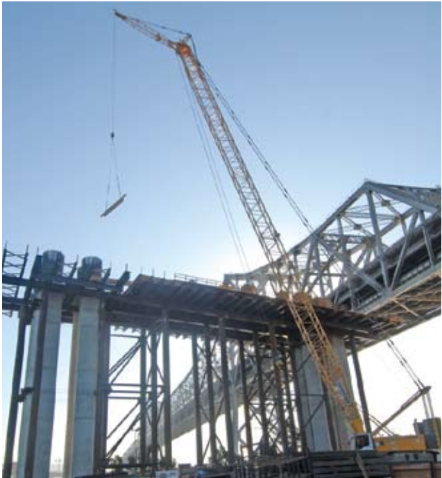
During the 2007 Labor Day Weekend closure, the bridge was closed in both directions to allow workers to replace a 350-foot section of roadway.
