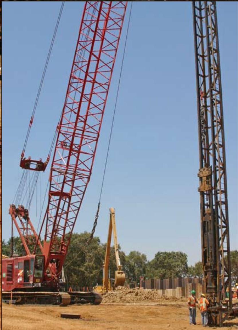
From left: Oiler Apprentice Jesse Rigby and Crane Operator Evan Trujillo prepare to drive pile for the Coon Creek overpass as Excavator Operator Von Marquez digs a coffer dam.
