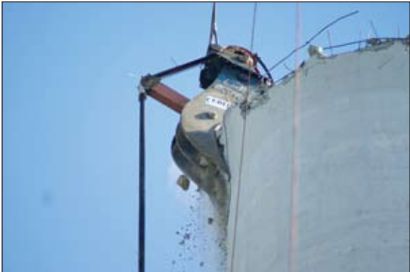
EBI uses massive jaws to break apart the Cowell Tower.
