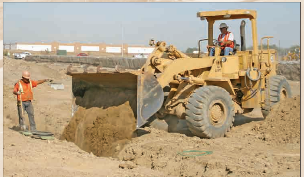
Operating Engineer Brian Evans, owner of B.D. Evans, unloads sand to insulate the underground pipeline.
