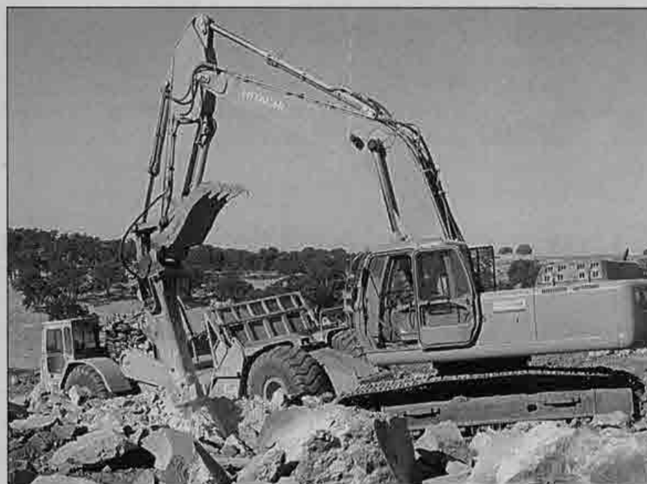
A hoe ram breaks up surface rock before scrapers take charge of the area.
