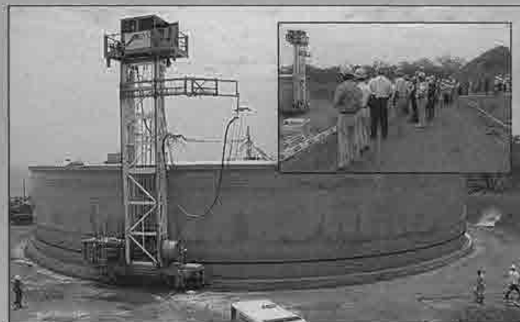
Operating Engineer Brett Crockett runs the pre-stress wire-wrapping machine on the two-million-gallon water reservoir being constructed by DYK in Kona, Hawaii. Oiler Joseph Pacheco Jr. and Crane Operator Russell Hall also work at the site. Inset: Contractors and county personnel watch the wire-wrapping machine in action at the DYK worksite July 24.
