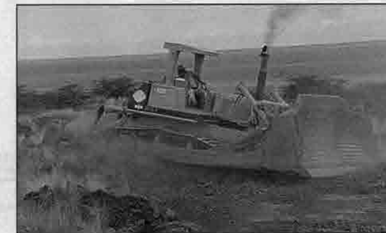
Above: Harry Medeiros works on the 275 Dozer.
