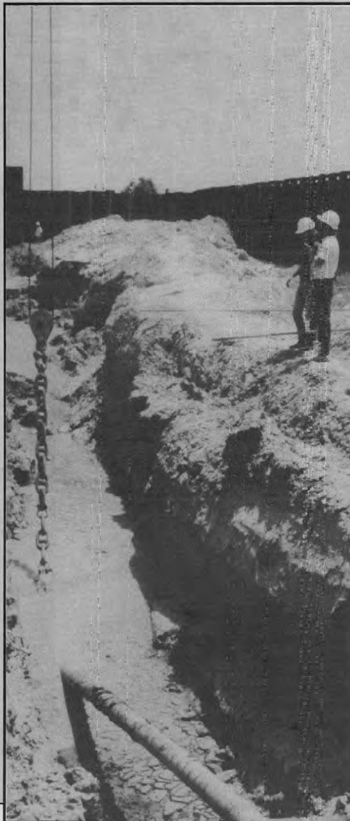
Top: X-ray technicians make last-minute weld inspections just prior to the pipe pull-through at Dutch Slough.
