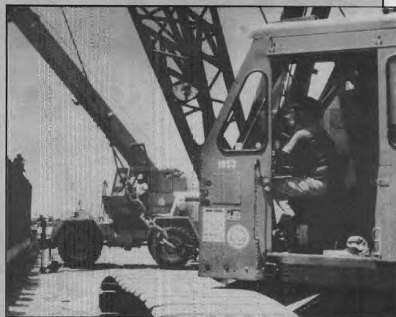
Above: A 100-ton Link-Belt LS 338, foreground, and a Grove CRT-183 were used to lift the pulling cable into position so it could be attached to the flex joint.
