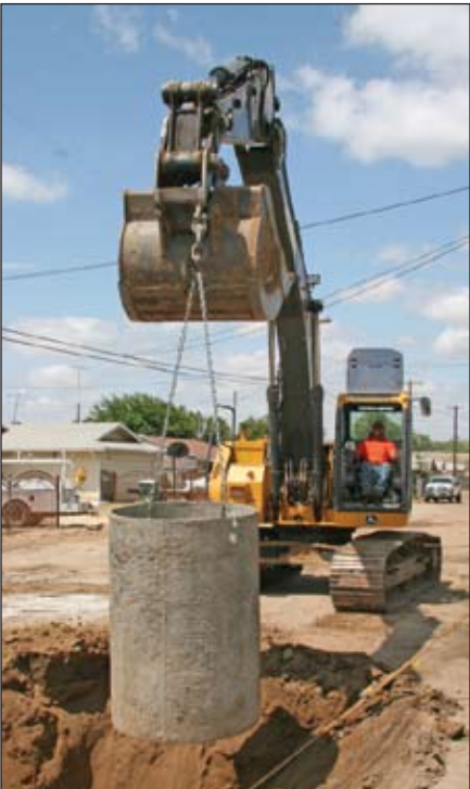
Excavator Operator Danny Everhart puts in a storm drain for Mozingo.
