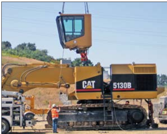
The CAT 5130 is assembled at the Folsom Dam jobsite.
