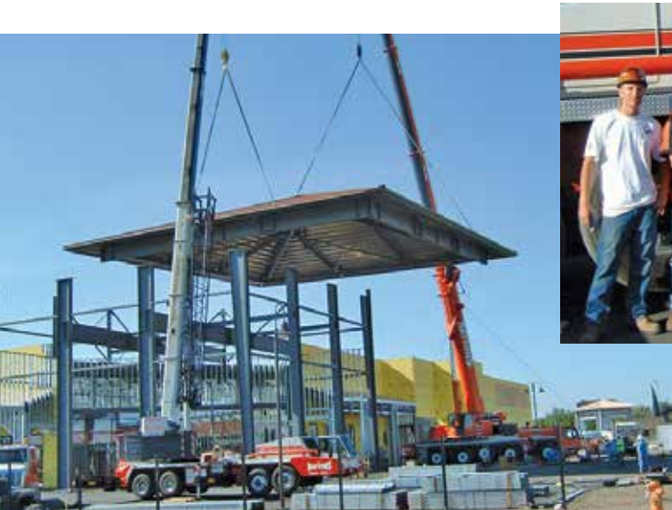
Working for Hatton's Crane , crane operators Troy Reese , Tom Hopken , Jacob Mendonsa and Abe Padilla use a 265-ton crane and a 90-ton crane to make a 56,000-pound lift for the new Harley Davidson dealership in Lathrop.
