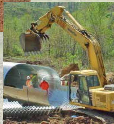
Member Kenny Spliethof assembles a multi-plate culvert for Steve Manning Construction.
