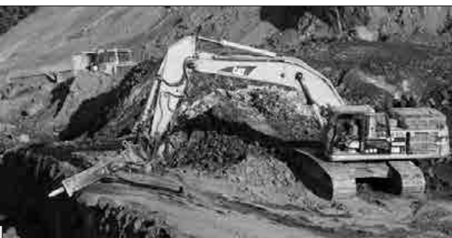
Member Robert Lee operates the hydraulic hammer excavator to break up large chunks of rock to be moved to the hillside below. Most of the land movement on the hilltop will make way for some 1,600 homes.
