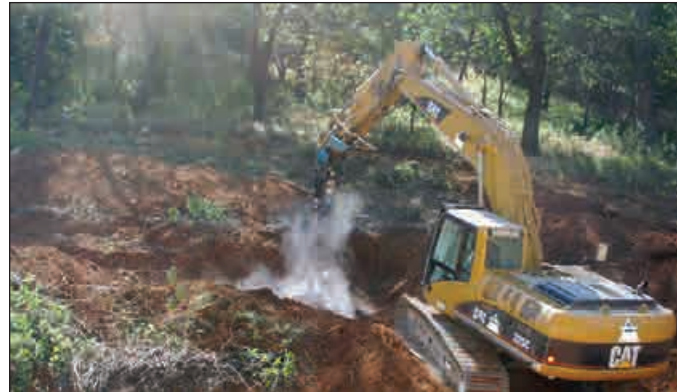
Local 3 member Bob Spence runs an excavator with a hydro hammer to break up a large boulder where the crew is clearing a hillside at the Lehigh Quarry.
