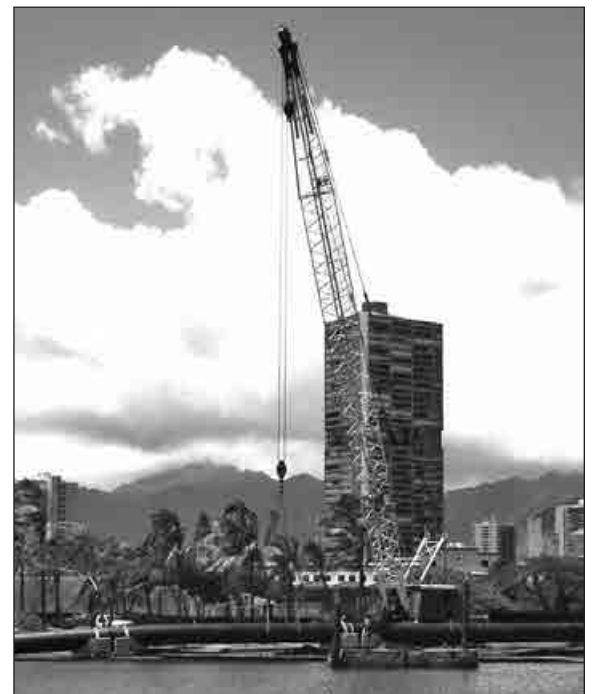
Members working for subcontractor Healy Tibbitts weld and lower 42-inch line into the Ala Wai Canal on the Beachwalk Sewer Bypass Project.
