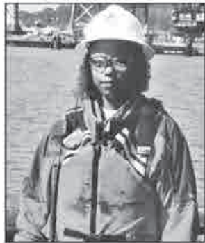
First-step Apprentice Bree Demings works for Kiewit's joint-venture on the Skyway portion of the Bay Bridge. This is the first time she has worked near water.
