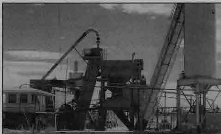
The vintage 4,000-pound Mattson batch plant has worked hard since 1955.
