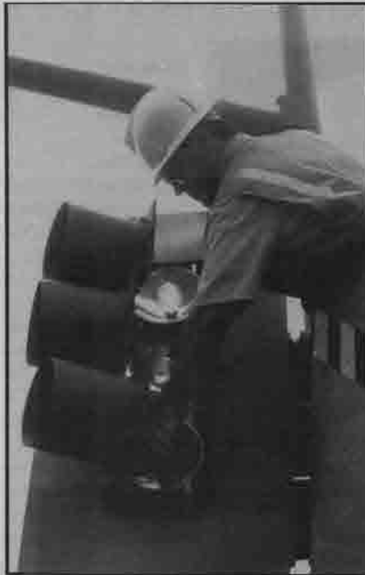
Above left: Victor De La Cerda replaces signal light bulbs before they burn out and cause a traffic hazard.
