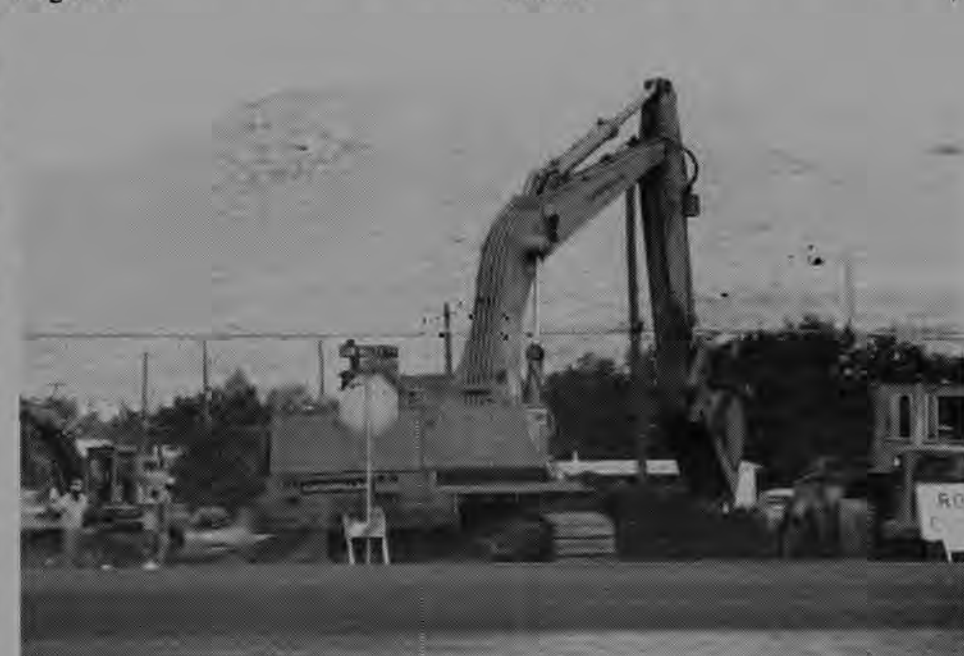
The H.M. Byars construction crew works on installation of 26 miles of 8-inch sewer lines for Sun Valley water and Sanitation District.
