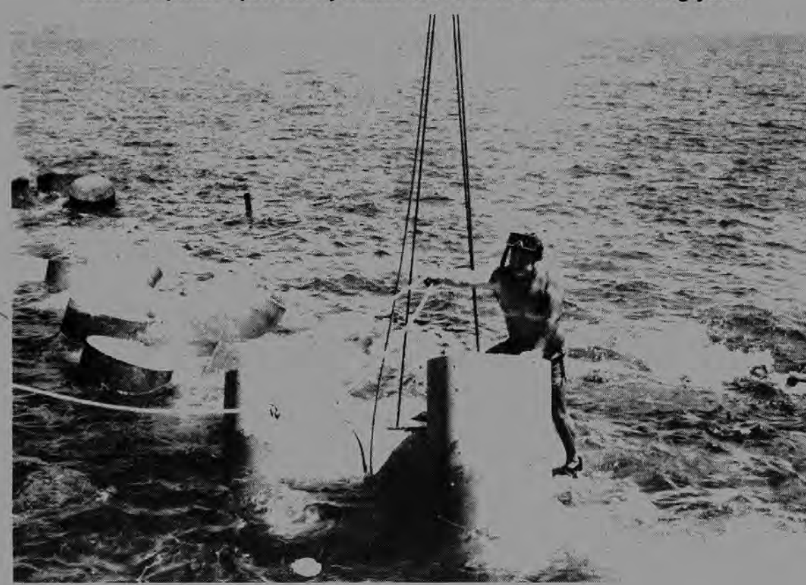
Brother John Kamoku sets tribars for the Hilo Breakwater project.
