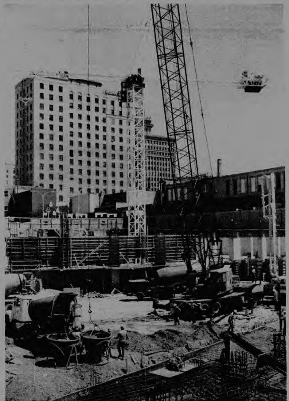
One of the largest continuous concrete pours in the history of Utah construction took place last month as workers laid the foundation to Salt Lake City's American Plaza III office and hotel complex. For more photos and story, see page 8-9.
