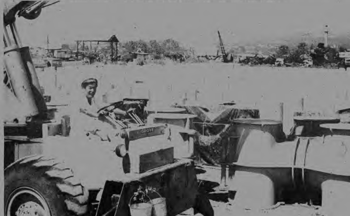
Ichiro Fujimori operates hydraulic crane in the Bohemia casting yard.
