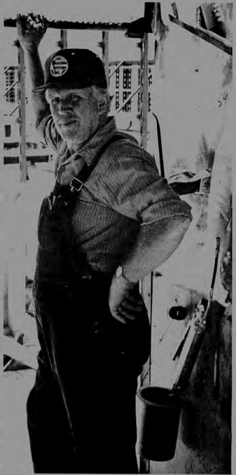
Sven R. Renning, elevator operator at Marriott Hotel job.
