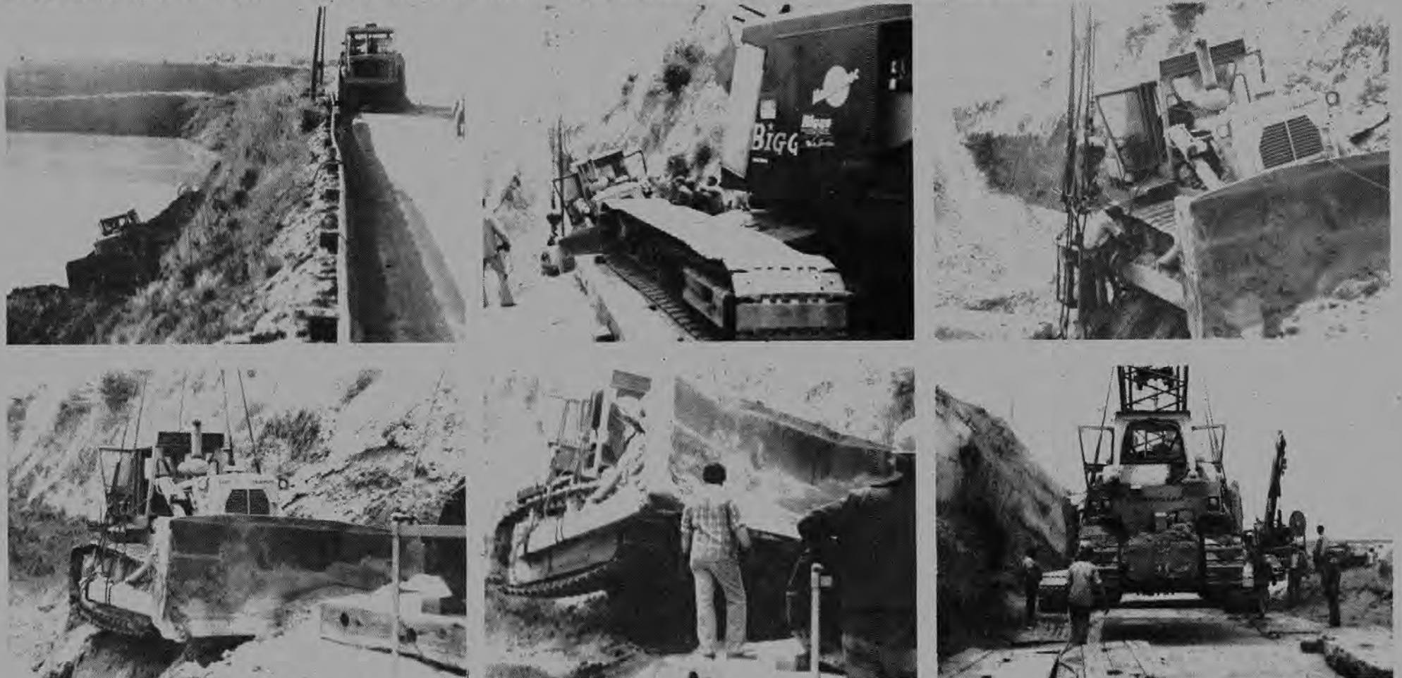
Starting from upper left, scraper ties off dozer, crane prepares the pick after workers hook cables and the lift is made to safe ground.
