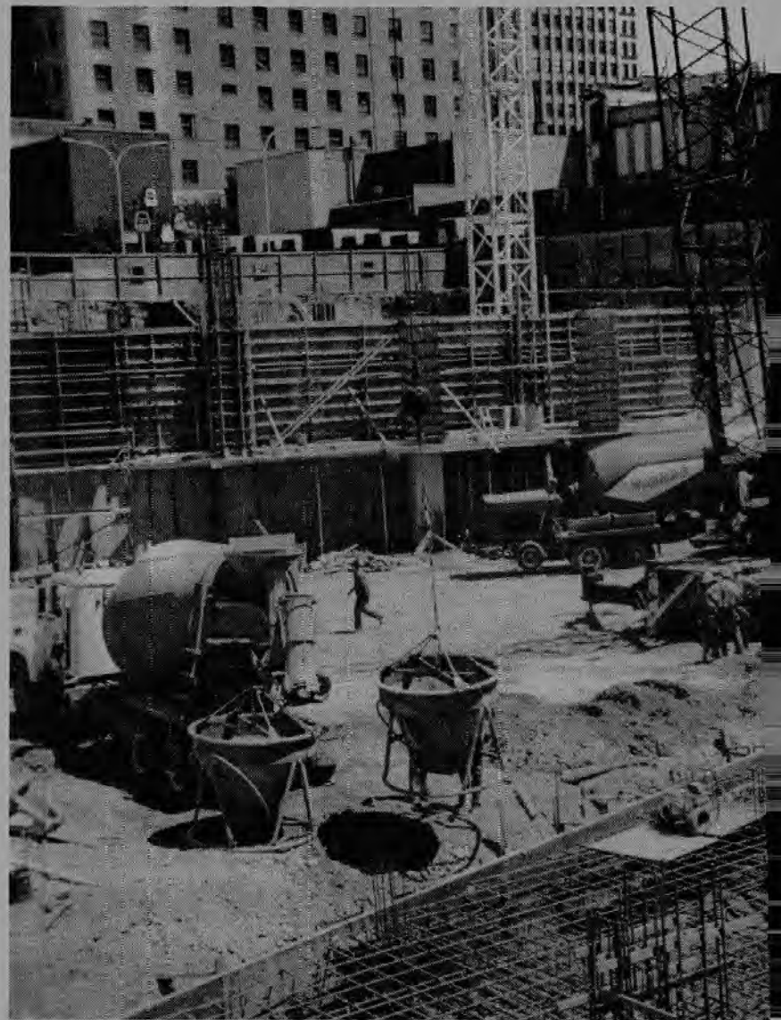
Pictured above and below is the high concrete pour recently
