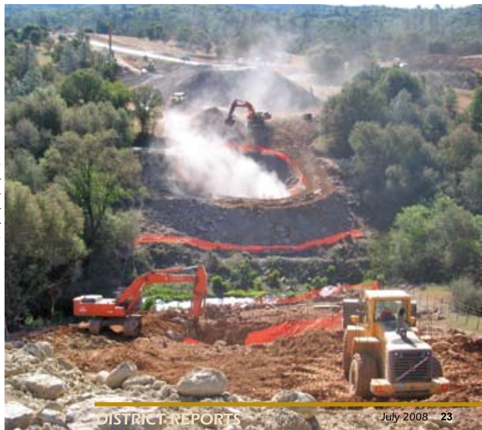
MCM Loader Operator Elias Madrigal and excavator operators Wayne Dahlquist and Bob Ryan dig the pier footings for a bridge over Angels Creek on the Angels Camp Bypass.
