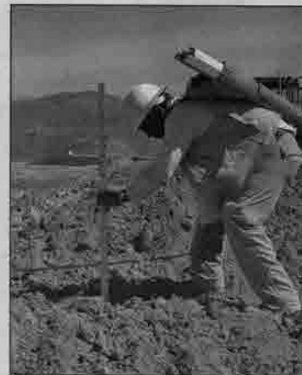
Gradechecker and 30-year Local 3 member Ted Sanchez places a gradestake on newly leveled ground on Phase 4.
