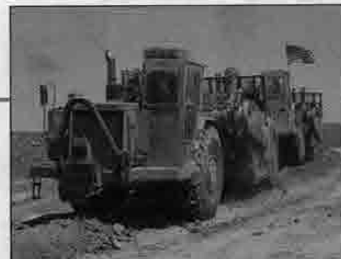
A scraper pushes dirt downhill on the Windemere side of Dougherty Valley near San Ramon, Calif. .... 4
