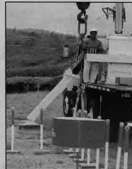
Hawaiian Dredging & Construction's Noa Nakoa on the boom truck.
