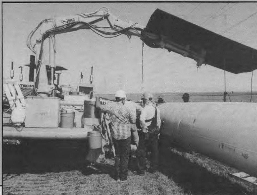
Top: Sidebooms prepare to lower sections of pipe along H.C. Price's spread north of Redding.
