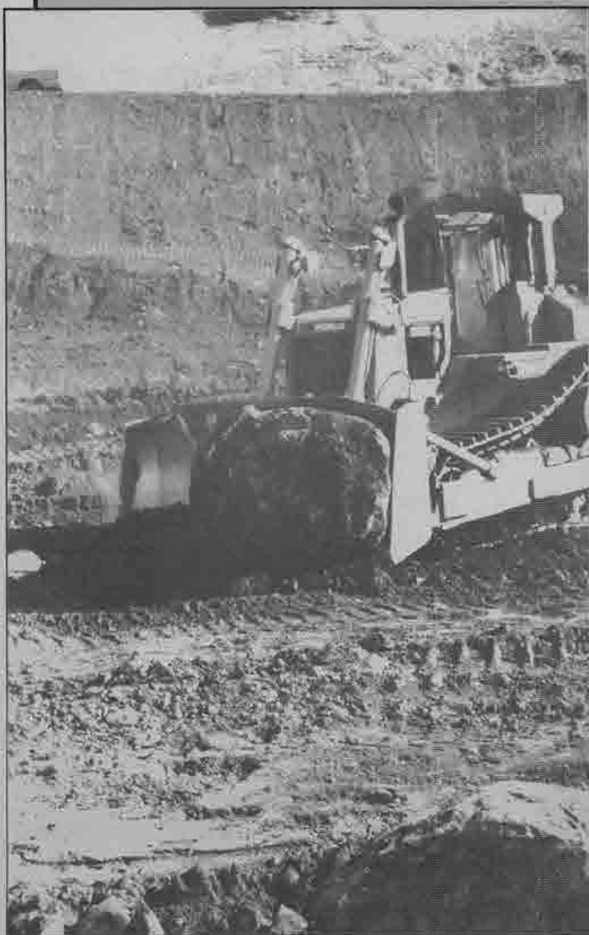
Huge boulders uncovered by the dirt moving operation (above) are moved out of the way by a crew of dozer operators. Below are Local 3 Business Agent Ted Lyman (left) and foreman Sonny Kemp, a 24-year member.
