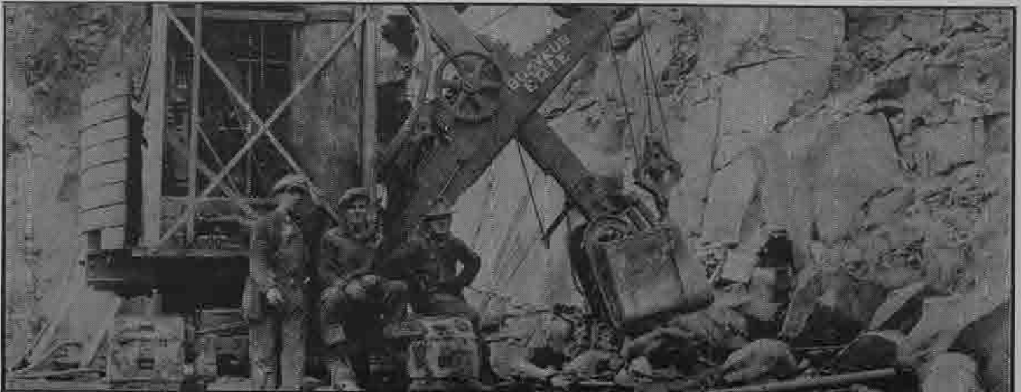
This old shovel helped bore the 11/4-mile Zlor-Mt. Carmel Highway tunnel in 1927. The operator was Whitney Erickson of Cedar City, Utah, and the offer was Local 3 retiree Bud Dalton, who was only 13 years old at the time.
