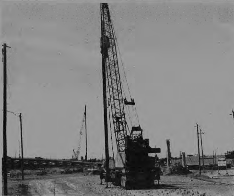
One of the many major highway construction projects that received heavy support from Local 3 is the Hwy. 101/92 interchange in San Mateo. After years of delay, this $40 million project is finally underway. The new project will relieve traffic congestion by providing four lanes in each direction on Route 92 and reconstructing portions of the interchange.
