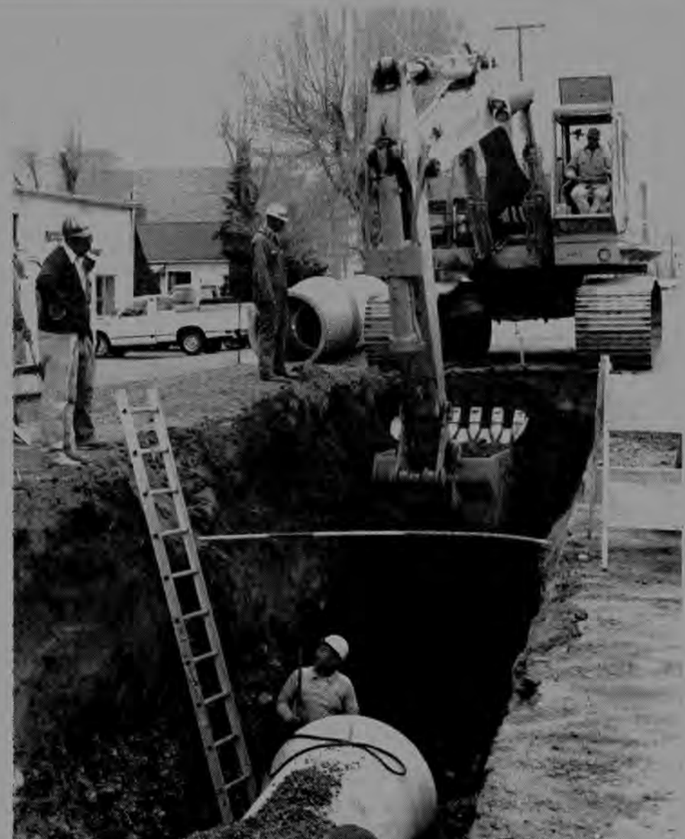
Pictured above is the cross-town interceptor job in Reno. R.L. Helms is the general contractor.
