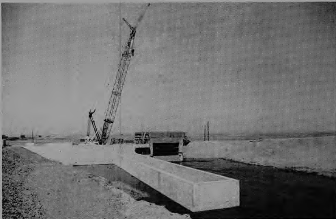
Currently under construction and due for completion this October is Turlock Irrigation District's small hydro-electric power plant on the Merced
