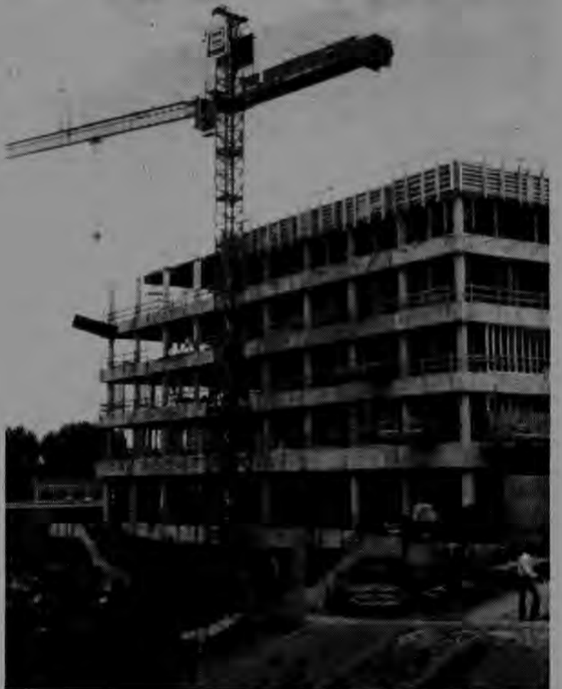
Pictured above is the University of Nevada's new 7-story college of business administration currently under construction at a cost of $6.2 million. Walker-Boudwin is the general contractor.
