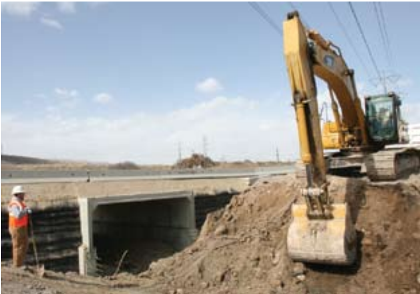
Bryson Ashworth watches Excavator Operator Andy Gunther dig out an embankment for the third wildlife crossing.
