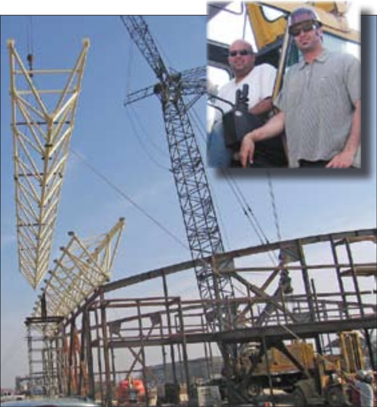
Mid State Steel Operator Bryan Gatschet and Oiler Vince Roseberry pick up a more-than-30,000-pound truss for the Gregori High School gym in Salida.
