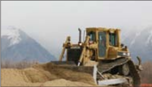
Sam McCurdy moves material to build an access road on the Pioneer Crossing project.
