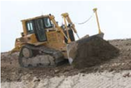
Brian Brunson cuts the slope to grade by adding top soil so it can be reseeded.
