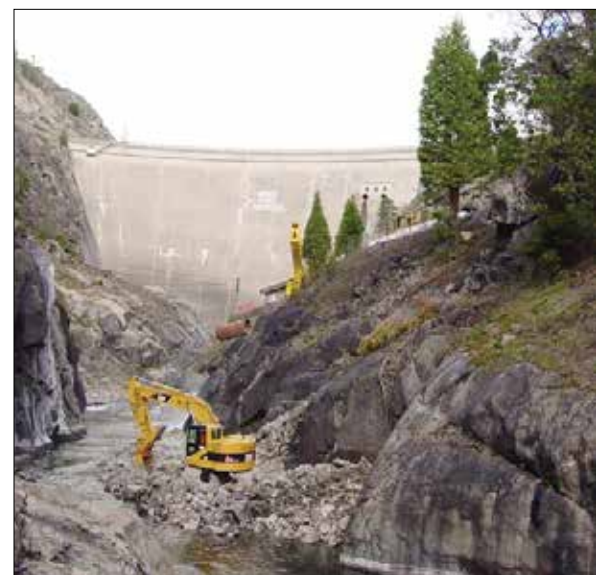
From left: Excavator Operator Caleb Johnson and Yarder Robert Sanders remove 8,000 tons of rock that slid down the vertical walls of the Tuolumne River Canyon at the O'Shaughnessy Dam. Johnson works for On-Grade Contracting, and Sanders works for Combined Effort.
