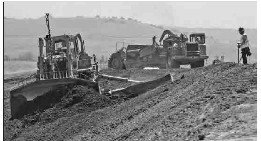
Gradesetter Ron Graves makes his marks for the scrapers in the field.
