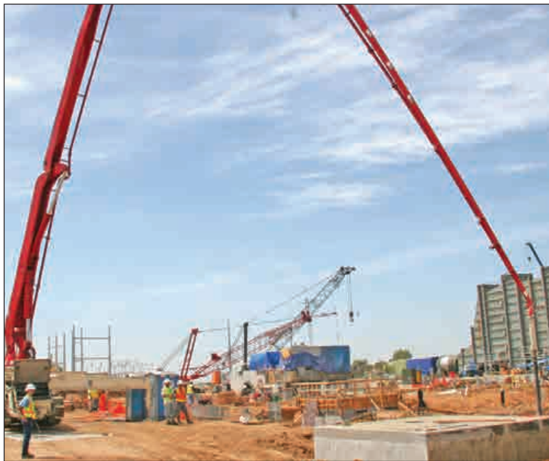
This 55-meter Putzmeister lays the footings that will hold a pipe as part of the new Roseville Energy Park.
