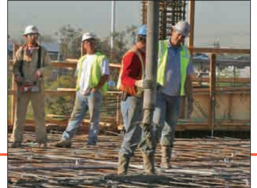
A 63-meter concrete pump is used to pour concrete for a new parking garage at Sac State. ....9
