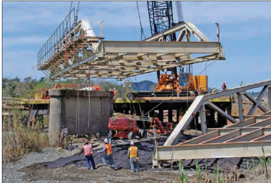
Members remove the bridge decking and dismantle the old Geyserville Bridge.
