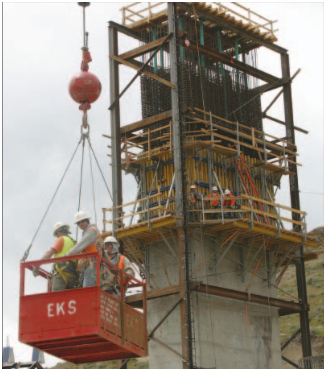
Crew members are transported in a manbasket by Crane Operator Mike Butler. They are working on one of 12 piers for the Galena Creek Bridge.
