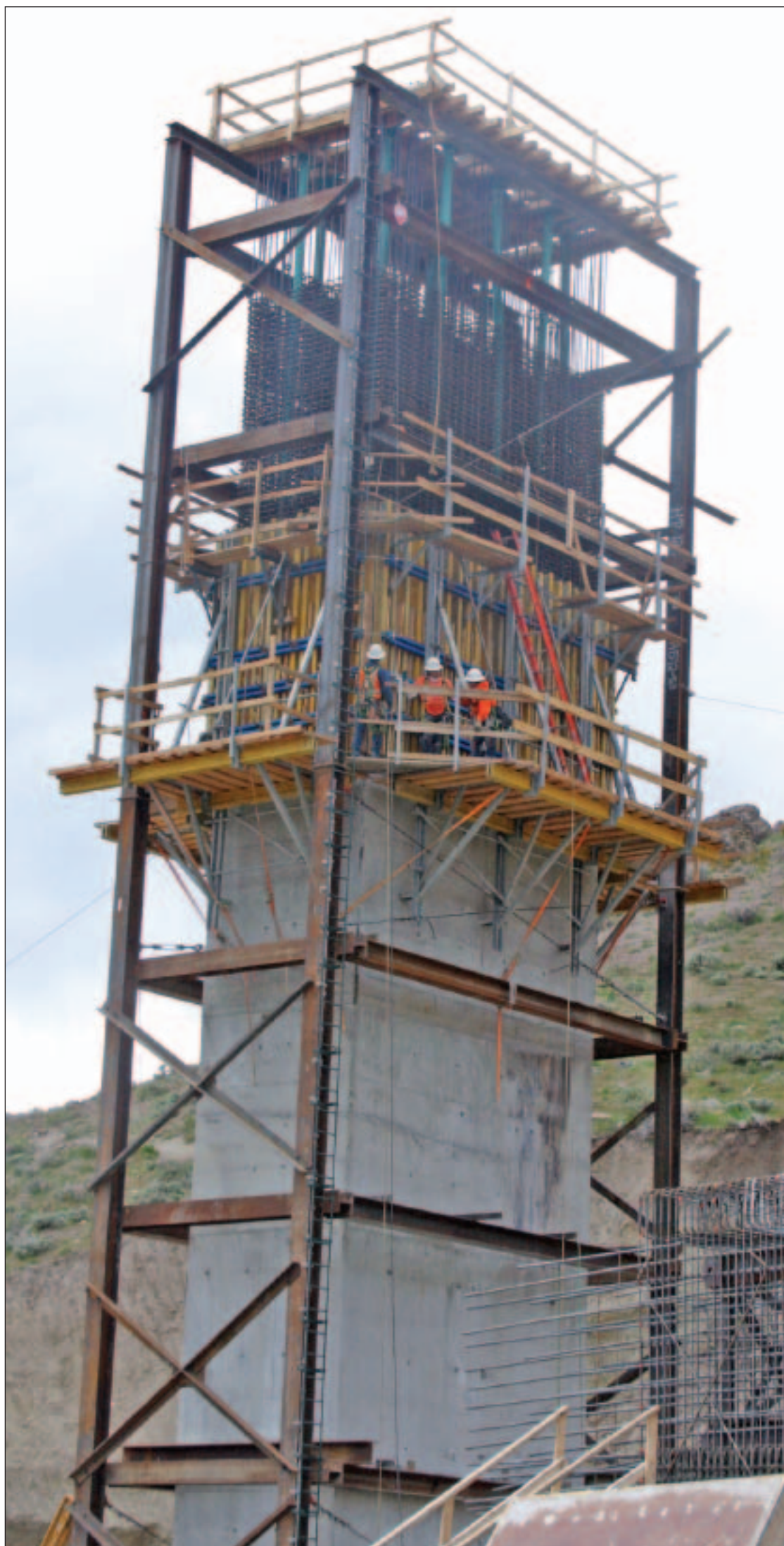
Local 3 members work on one of 12 piers for the Galena Creek Bridge at the I-580 Extension Project worksite in Nevada. With a 1,700-foot span, the bridge will be the longest of its kind in North America.
