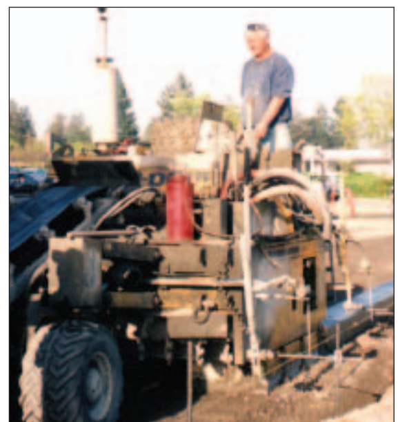
Local 3 Operator Doug Knoll pours concrete curbs and gutters in Rohnert Park for Arthur and Devinceni Concrete.
