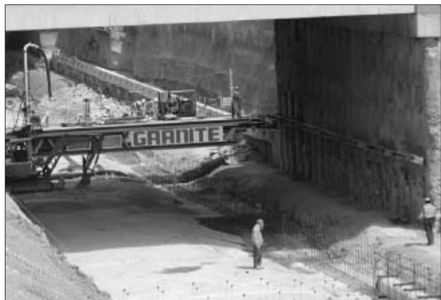
This trench is the site where the mainline tracks will be lowered to reduce the traffic and noise pollution in downtown Reno.
