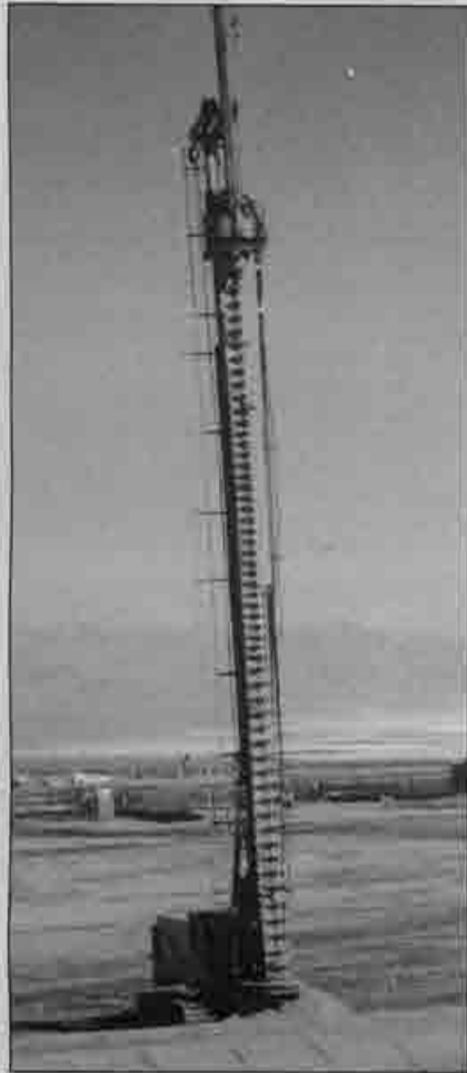
Using this drill, Geottle does foundation work in Mona, Utah, at the Currant Creek Power Plant project.
