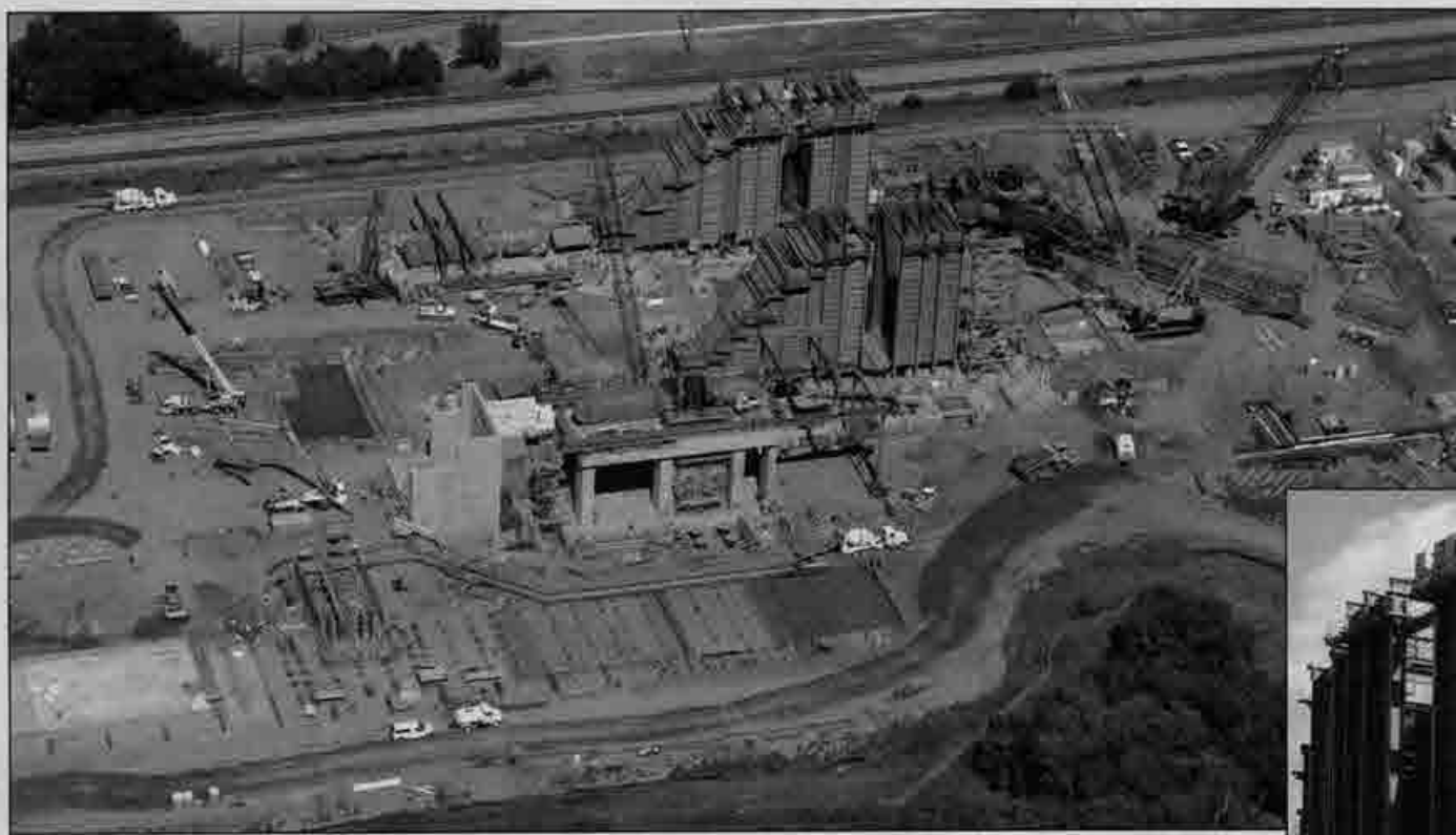
Above: An aerial view of the Metcalf Energy Center project from April 2004. (Courtesy of Calpine) At Right: The power plant will consist of two gas turbine generators, two triple-pressure Heat Recovery Steam Generators (HRSGs), one steam turbine generator, a cooling tower and a switching station. The HRSGs are made of 21 modules each. Four modules have been set into place. Two are shown here.
