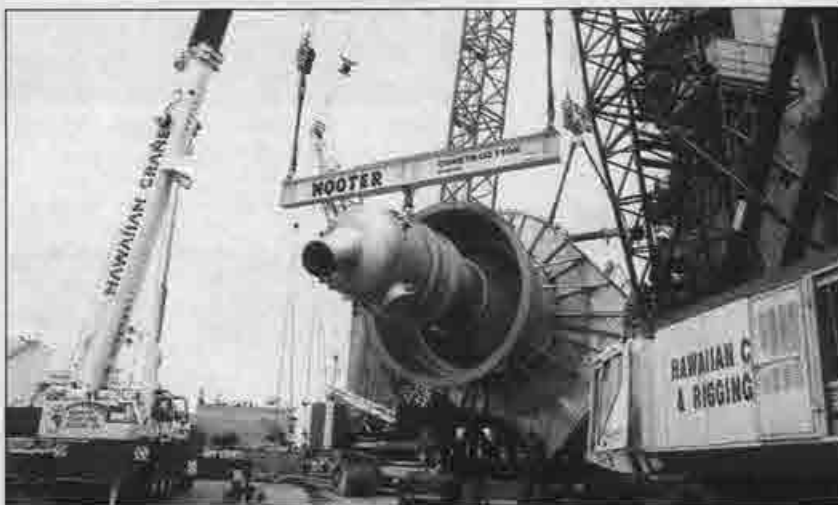
The three cranes lift the catalytic converter off the mobile transporter.
