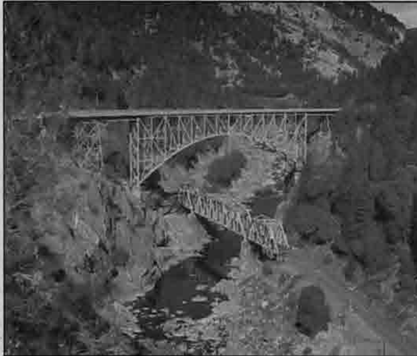
SCENIC VIEW: Hwy. 70 Pulga Bridge in Butte County north of Oroville on the Feather River was the recent site of a foundation exploration of both abutments and piers. A crew with a portable rig can be seen on top examining the historic two-lane bridge for a seismic retrofit that was later completed.
