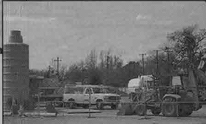
2. The large experimental fiberglass manhole used at the Rite Aid job is shown at far left.
