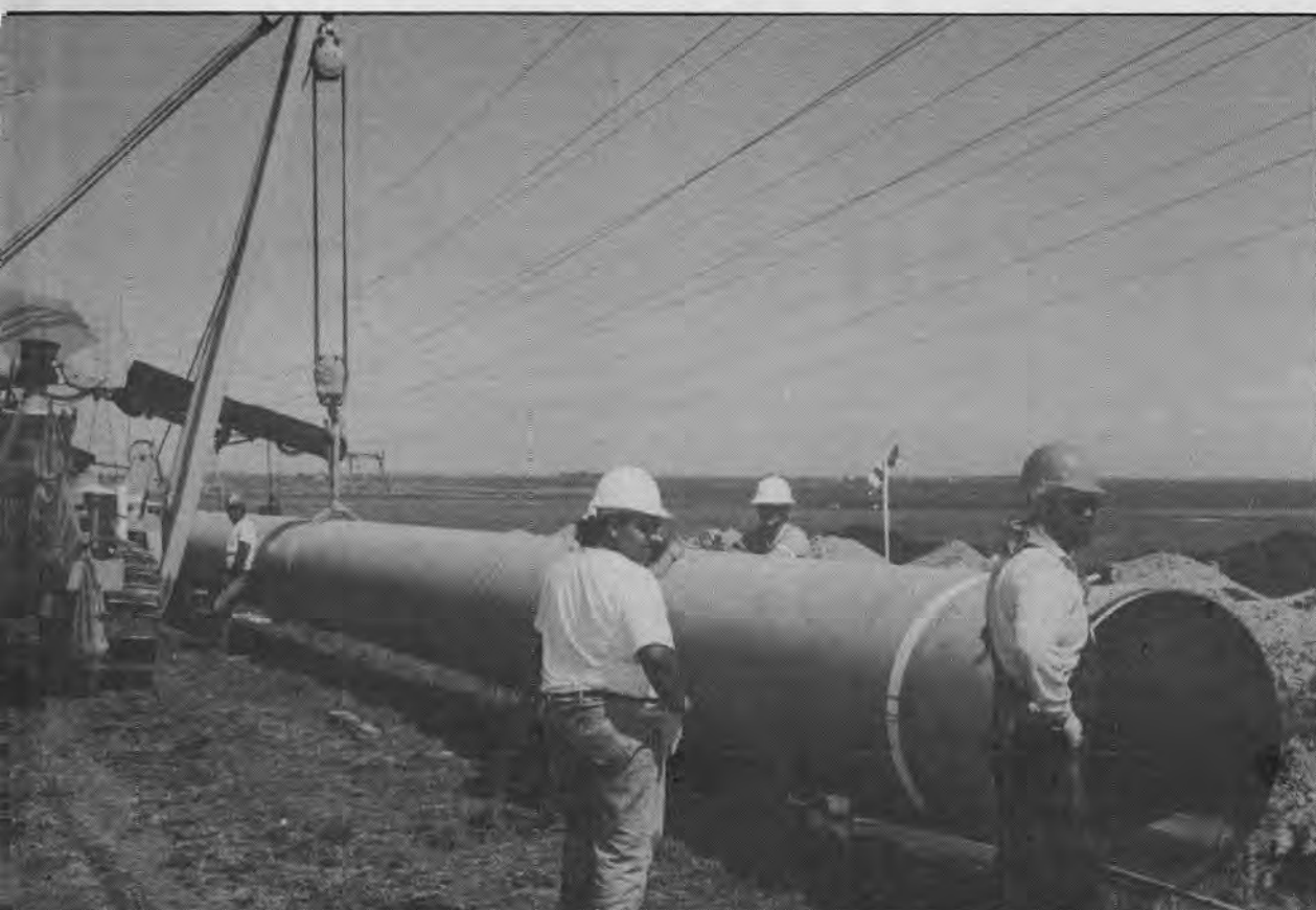
Left: A section of 42 - inch pipe is prepared to be laid on Spread 5.
