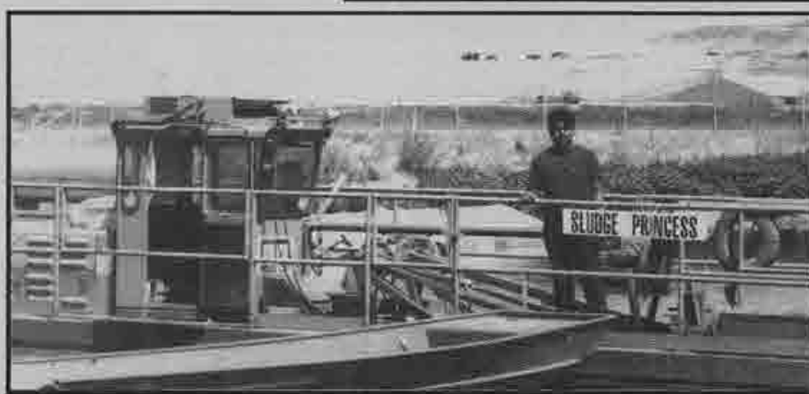
Above: Ken Dervell, operating a Brown Bear auger, churns up sledge so it dries evenly.
